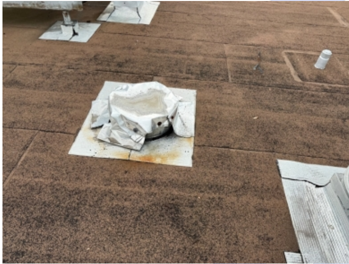
Improper Flashing
