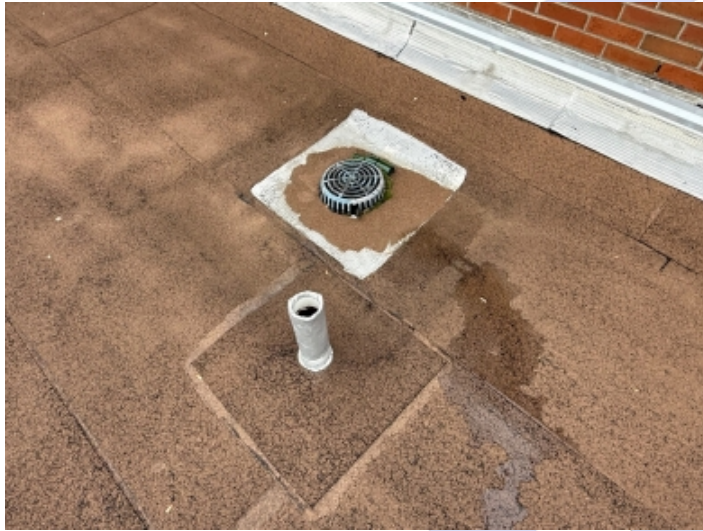
Debris & Granules in Drain Area
