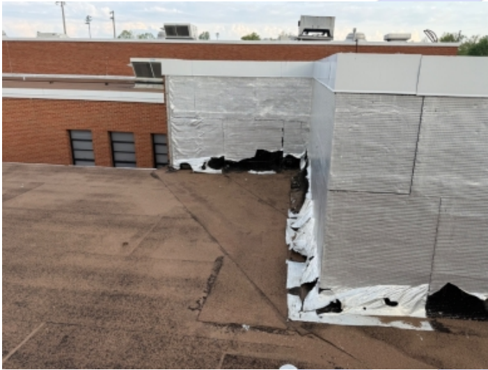
Wall Flashing Degradation
