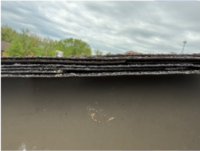
Multiple Layers of Shingle on Existing Structure
