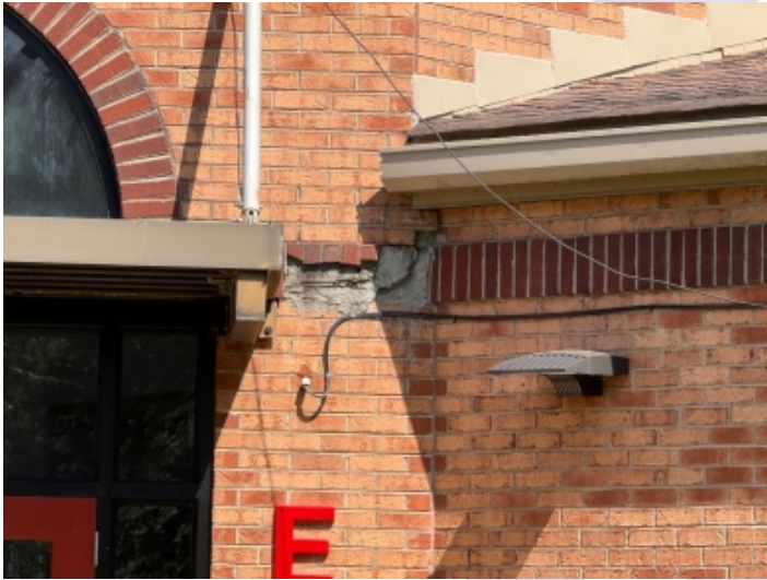
Masonry Cracking
