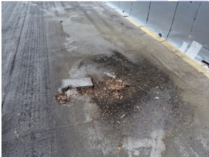
Existing Drain Clogged
