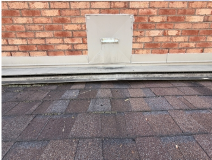
Scupper & Ventilated Headwall Flashing
