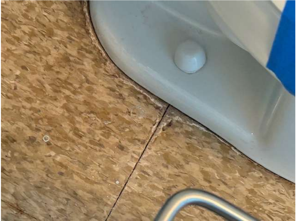
Water staining around the toilet.
