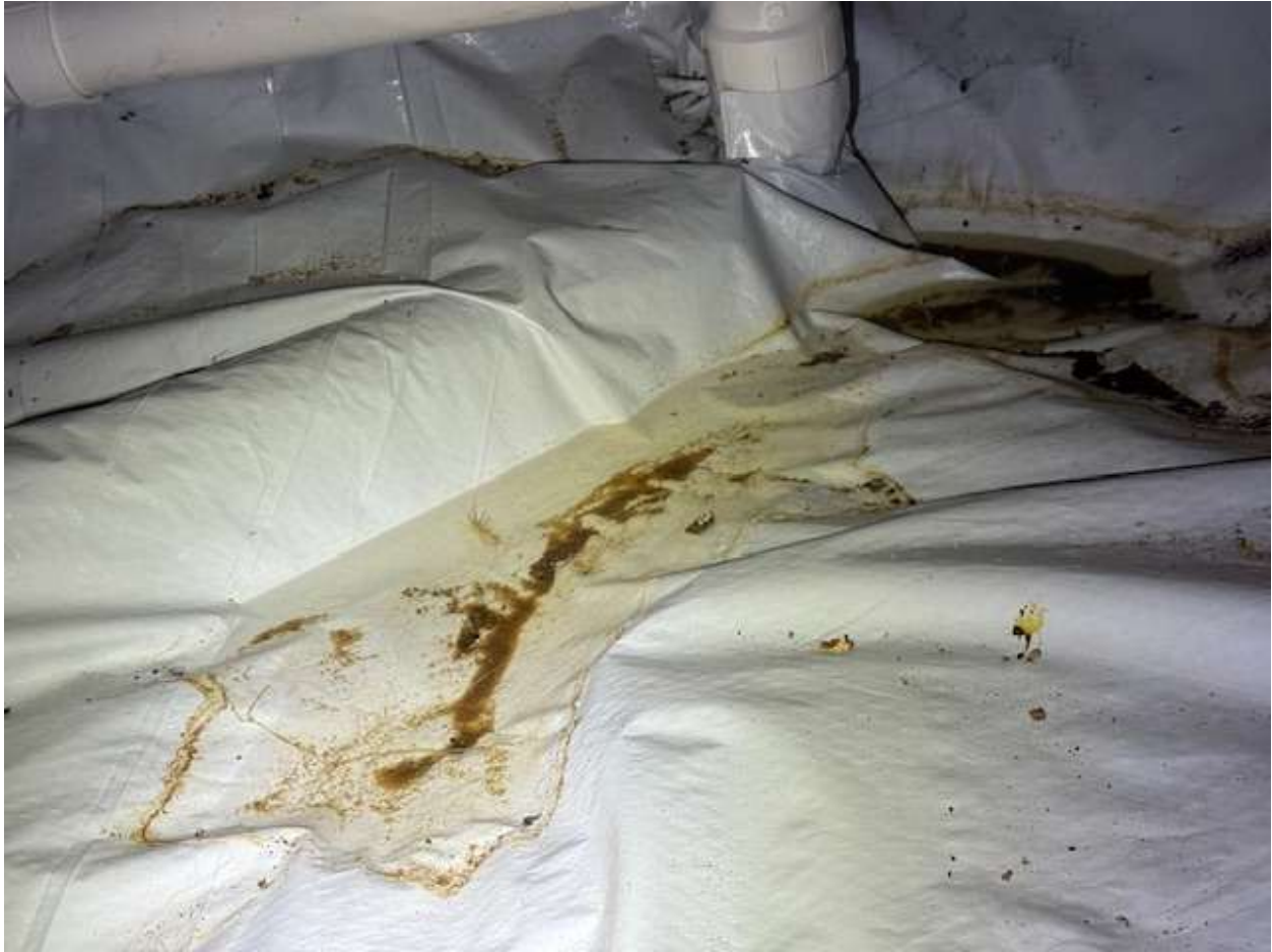
Standing water in the crawlspace under the affected area.
