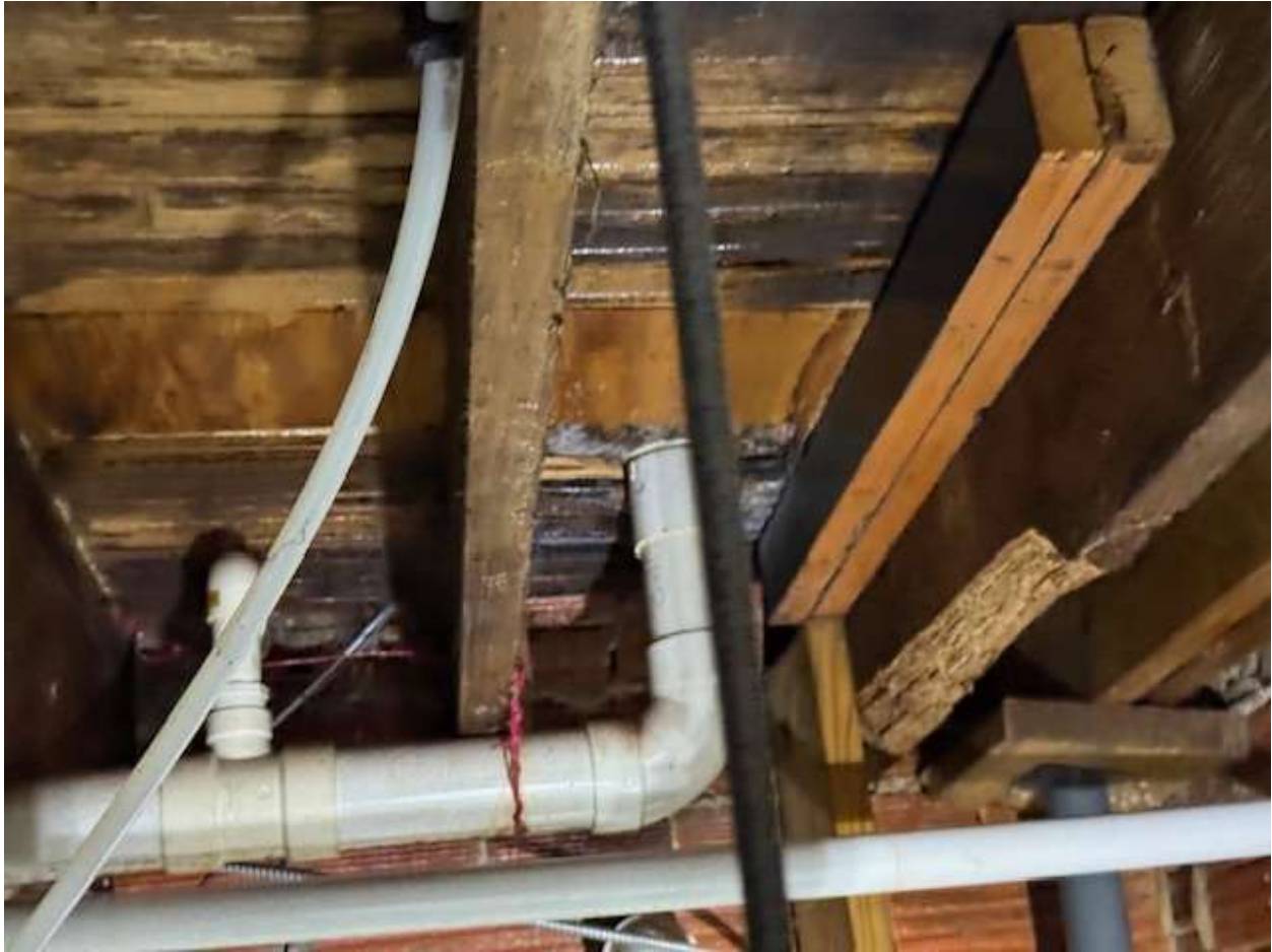
Underside of the subfloor. Water staining and mold growth are present.
