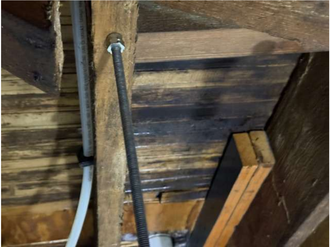
Underside of the subfloor of the affected area. Water staining and mold growth are present.
