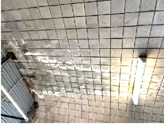
Water Intrusion in Library Stairwell
