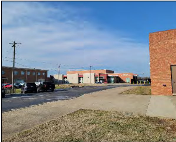
Photo 1. View looking northwest at building addition area.
