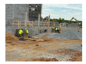
b) CMUs were being laid for the Gym/Storm Shelter. The walls appear to be nearing roof joist bearing elevations.
