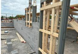
g) The Skudo system was being held in place with CMUs placed on top of the board.
