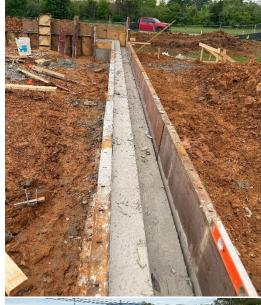
g) The under-slab plumbing piping for the toilets was covered with stone. Once the stem walls are poured, the plumbers will run the lateral lines in stone which will be covered with the concrete slab. Brad said that they will pour the slab before erecting the columns.
