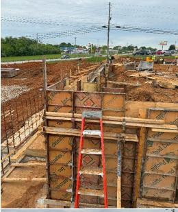
On the southeast corner of the office area, e) the ramp for access to the floor level was located by the dowels for the retaining wall. In front of this area paralleling Hwy 62 the site will contain the parking lot.
