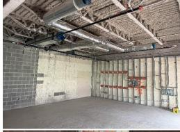
q) Floor slabs at new door openings on the second floor were filled with concrete. Floor prep will be required, but these areas appear to be properly prepared to receive floor finish,.
