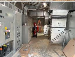
l) Hydronic piping and ductwork were being installed above ceiling in Area J on the first floor.
