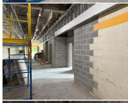
o) Metal framing and wallboard were properly installed to receive control joints in the soffits in Area J.
