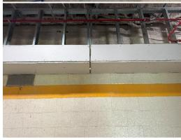
p) Where ductwork was installed the open ends were covered with plastic to keep dust out of the HVAC system.
