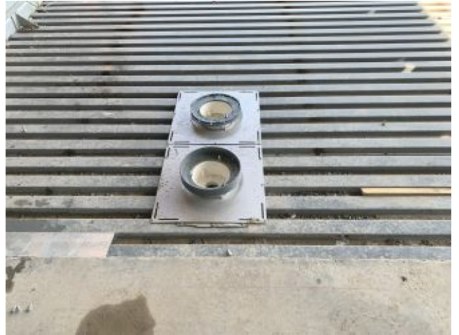
2025.04.01 – Roof drains at second floor patio
