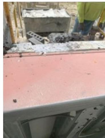
2025.04.09 – Missing liquid flashing at a first floor sill
