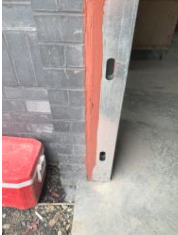
2025.04.15 – Air barrier repair at opening #121
