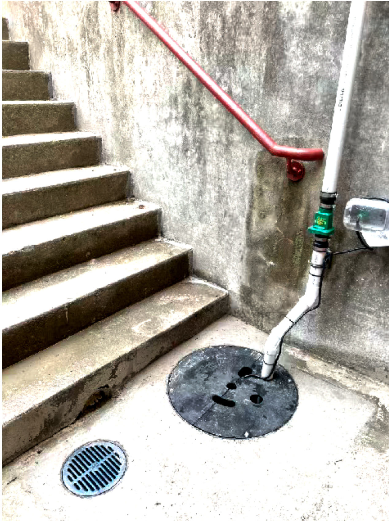
Sump pump drainage piping
