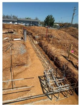
d) Steel reinforcement was in place at the northeast corner.
