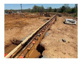
The footing on the southeast corner drops c) significantly to bear on suitable soils. The reinforcement that was in place reflects that. The footing bottoms appeared to be firm.
