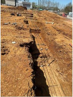
f) Soils were being removed to reach plan bottoms.
