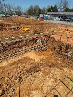
e) The footing steps to the southeast. Steel reinforcing was placed on concrete block risers.
