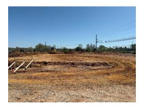
b) Some mud was washed onto the footings from the rains. The mud will need to be removed before the stem walls are added.
