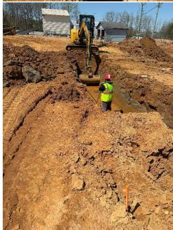
g) Once soils were excavated, it was removed to the area in front of the facilities building for loading onto dump trucks.
