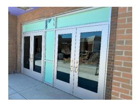
b) This storefront window was installed, but the metal window sill was not completely installed. The sill needs to integrated with the window frame so water is directed to the exterior.
