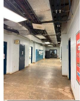
s) In the one story area, the asbestos abatement contractor has removed the asbestos containing floor tile and adhesives. They also removed the wall base.
