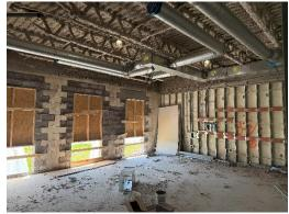
r) In the corridors in Area J, the lay-in ceilings have been removed. Gill reported that the contractors are indicating that space for above ceiling systems will be tight as they plan for the that work.
