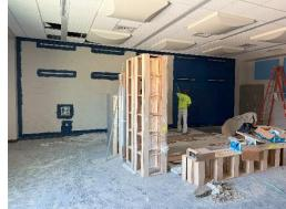
**k)** The wall above the overhead door for the band room was ready for the insulation and metal panels.
