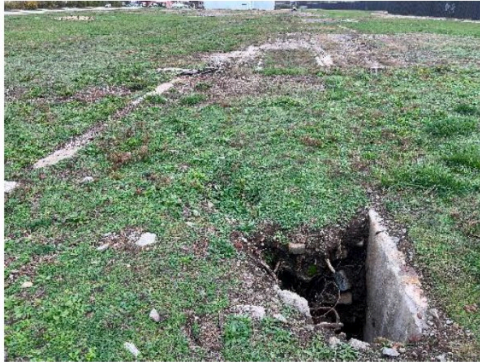
Photograph 2: Example of Backfilled Basement Encountered
