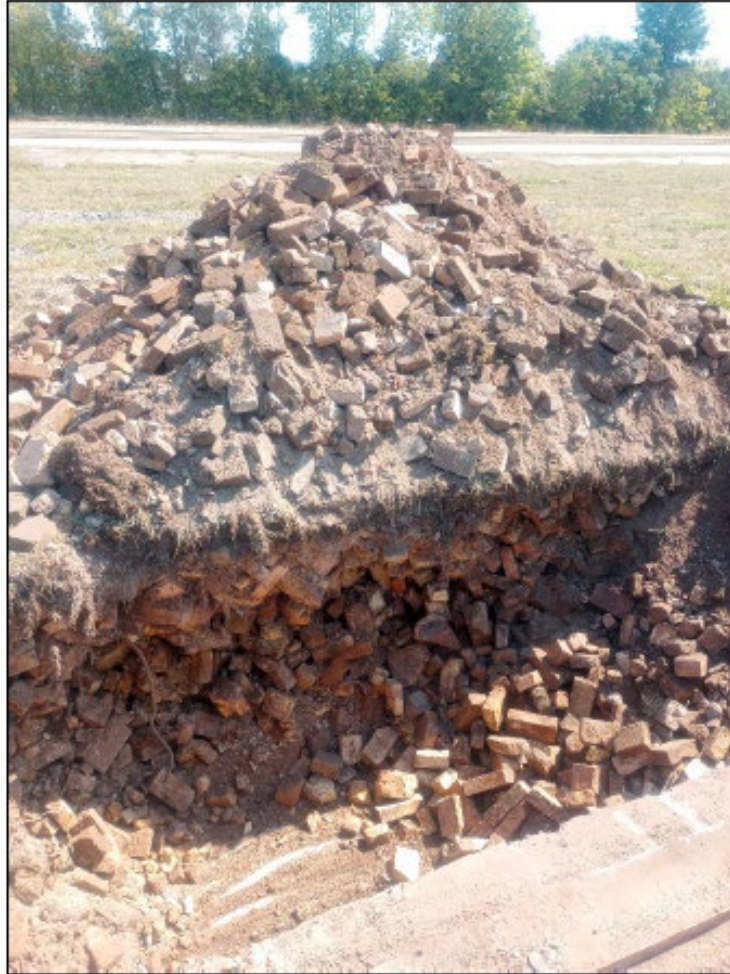
Completed Test Pit
