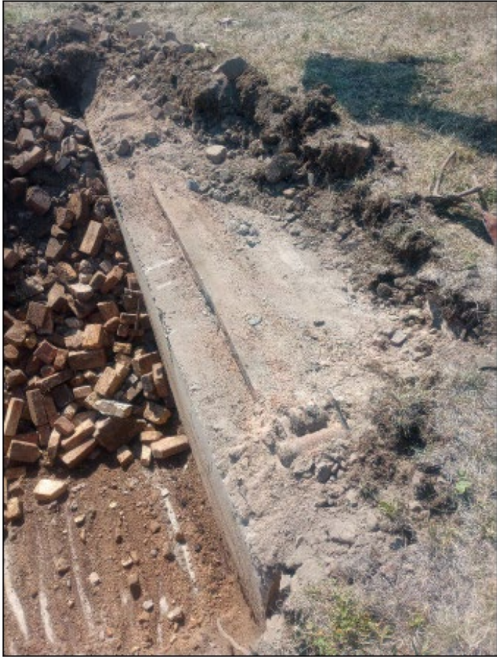
Large Buried Concrete Base with Steel Rail and Pulley's
