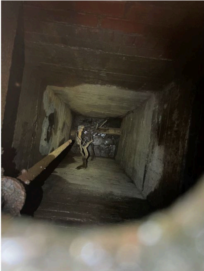
Photograph 8: Inside of Underground Shaft (UGS)
