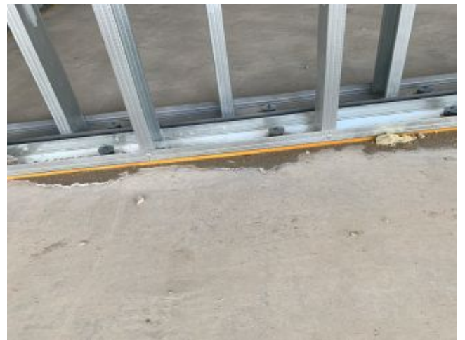
2025.02.07 – Sound isolation board at bottom of Production Studio wall
