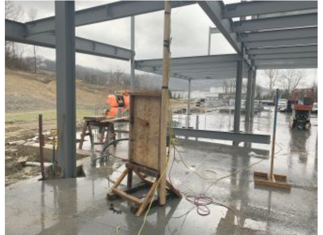
2024.12.10 – Temporary electric in Kitchen/Breakroom #165
