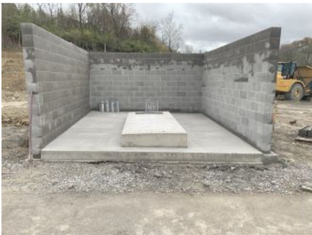
2024.11.06 – Generator screen wall
