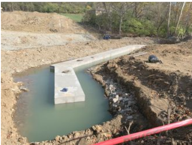
2024.10.29 – South footing for arch bridge
