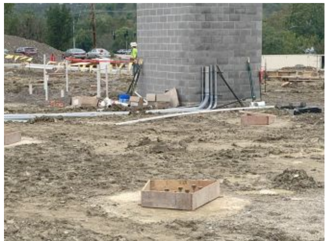
2024.10.01 – Electric rough-in at elevator shaft
