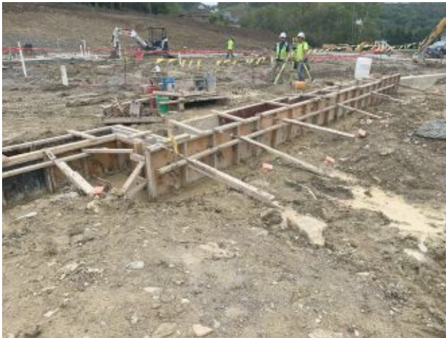
2024.10.01 – Foundation formwork at future entry
