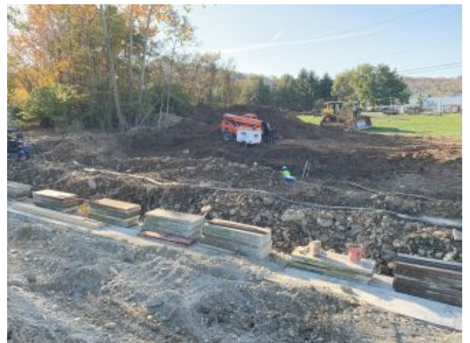
2024.10.23 – North bridge footing in foreground, south footing excavation beyond
