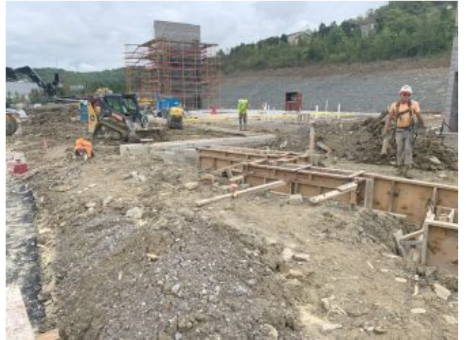
2024.10.01 – Foundation formwork at the sawtooth
