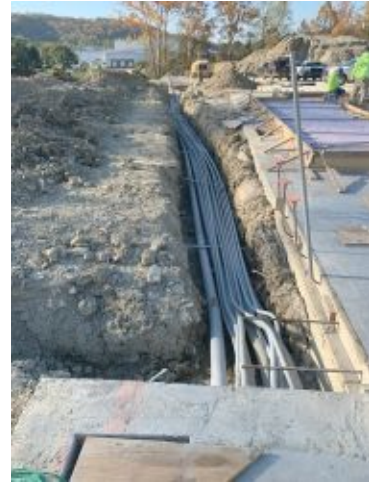
2024.10.23 – Electric conduits along east end (exterior) of Board Room.
