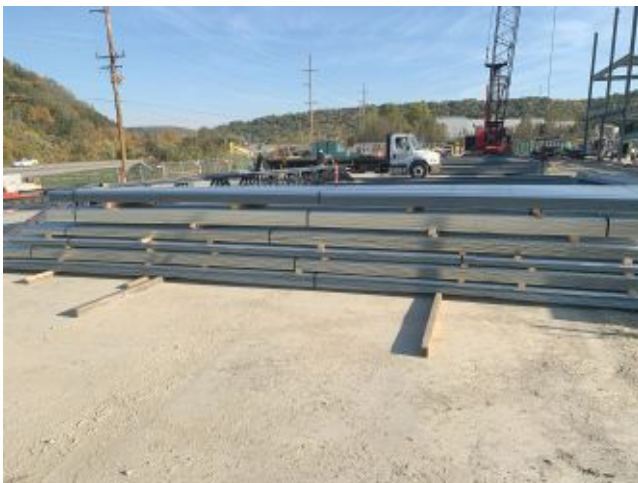
2024.10.23 – Galvanized deck for elevated slabs
