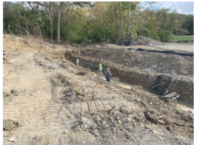
2024.10.15 – Bridge footing excavation
