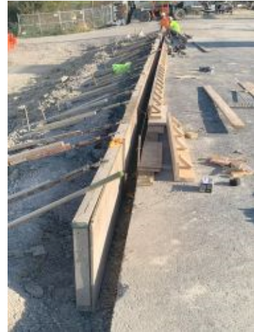
2024.10.23 – Header curb being formed
