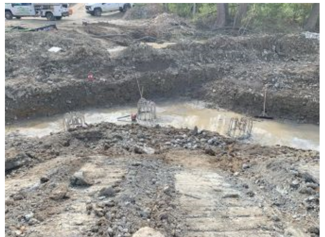
2024.10.15 – Bridge footing excavation
