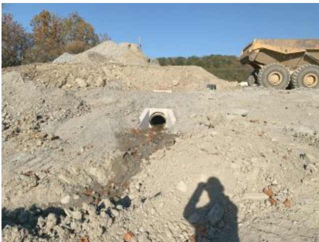
2024.10.23 – Headwall at future detention basin
