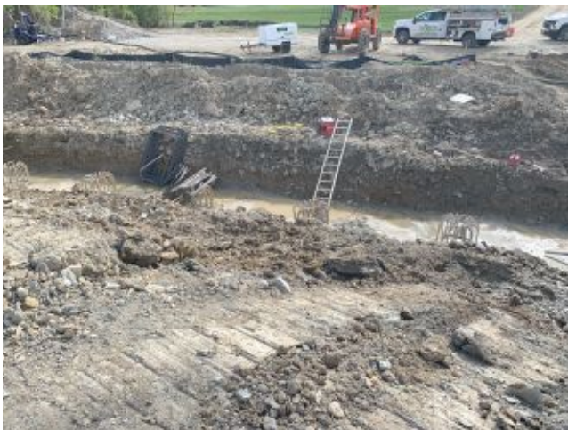
2024.10.15 – Bridge footing excavation
