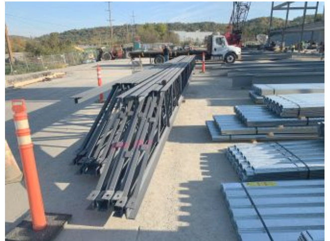
2024.10.23 – Board Room roof long-span joists
