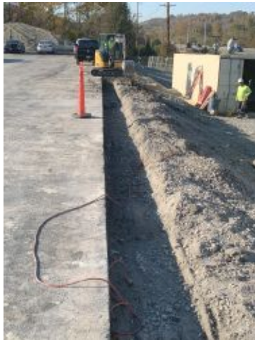
2024.10.23 – Header curb excavation
