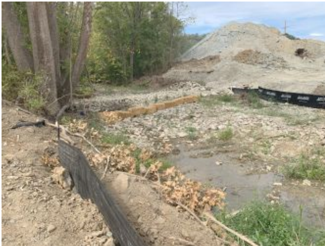
2024.09.17 – Construction waste containment across creek.
