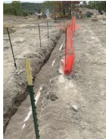
2024.09.03 – Underslab sanitary Area B, looking south.
