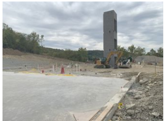
2024.09.17 – Completed masonry elevator shaft.
