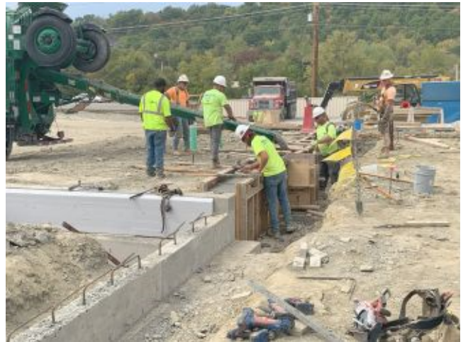
2024.09.17 – Pouring foundation along Line 0.8.
