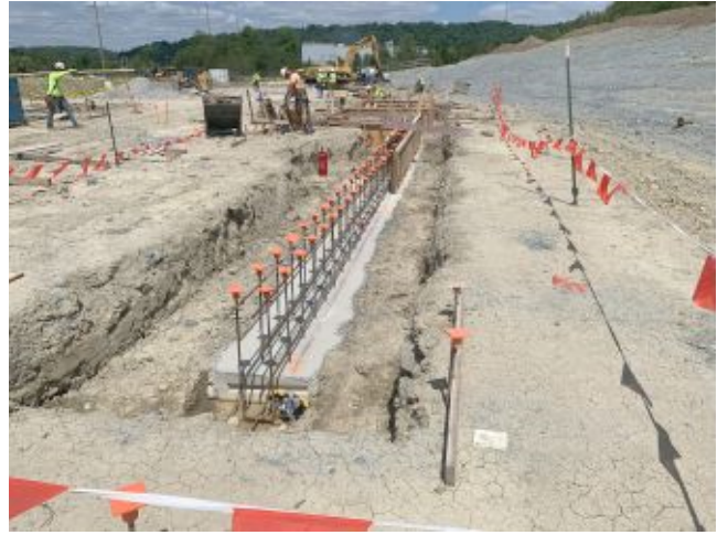
2024.08.20 – Footing along line F.
