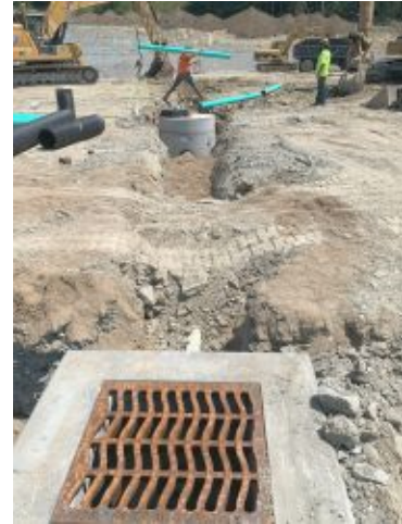
2024.08.06 – Storm structures #9 and #13.
