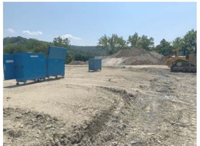
2024.08.06 - Building pad looking south/southeast.
