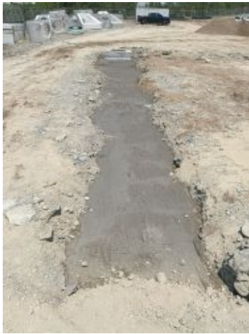
2024.08.06 – Looking towards storm structure #10.
