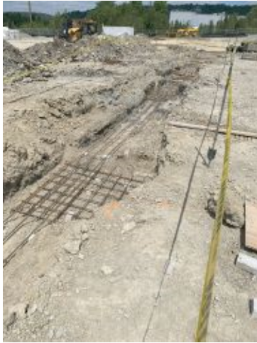
2024.08.20 – Excavation along line A.9.
