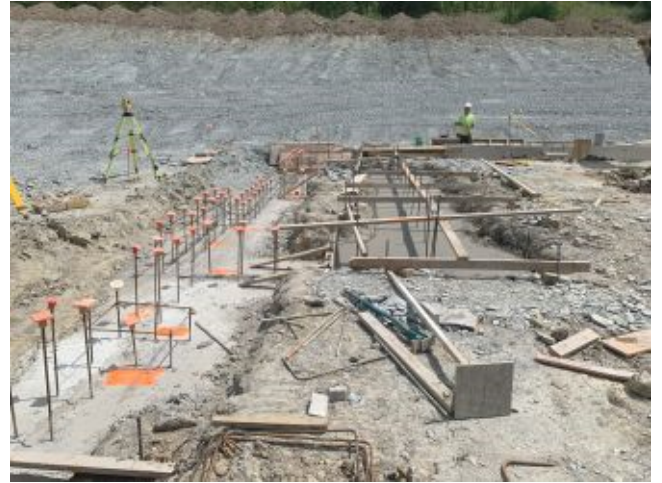
2024.08.20 – Line 11.1 and Stair S-1.
