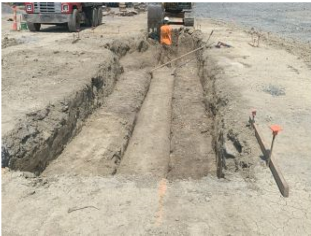
2024.08.06 – Start of footing/foundation at line F.
