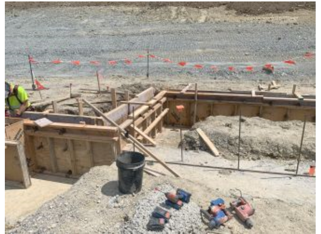
2024.08.20 – North wall of Stair S-2.
