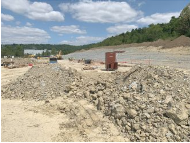
2024.08.20 – Looking north towards (E,11).
