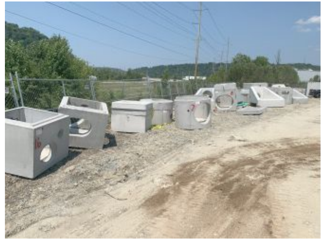
2024.08.06 – Storm structures staged for installation.
