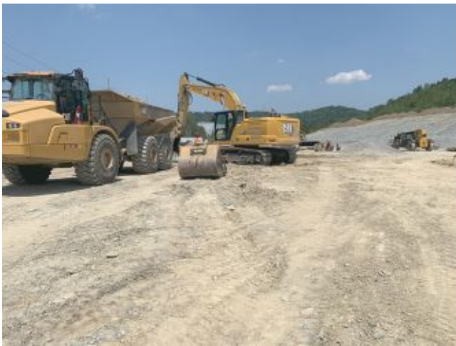
2024.08.06 – Building pad looking north.
