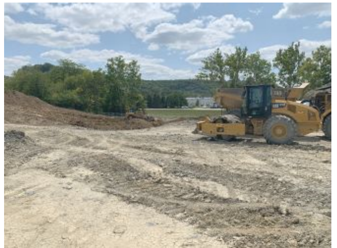
2024.08.20 – Looking towards future arch bridge.
