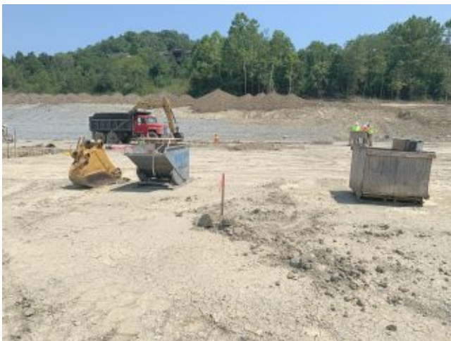
2024.08.06 – Building pad looking east.
