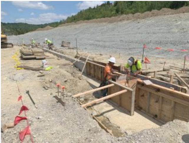
2024.08.20 – Foundation and formwork along line E.
