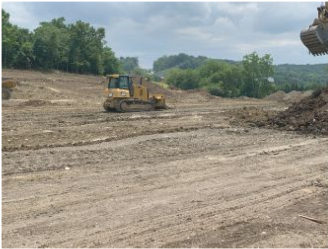
2024.07.09 – Site looking southeast.
