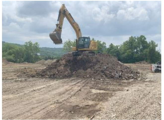
2024.07.09 – Site looking south.
