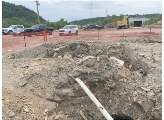
2024.06.26 – Basement under demolished wood structure.
