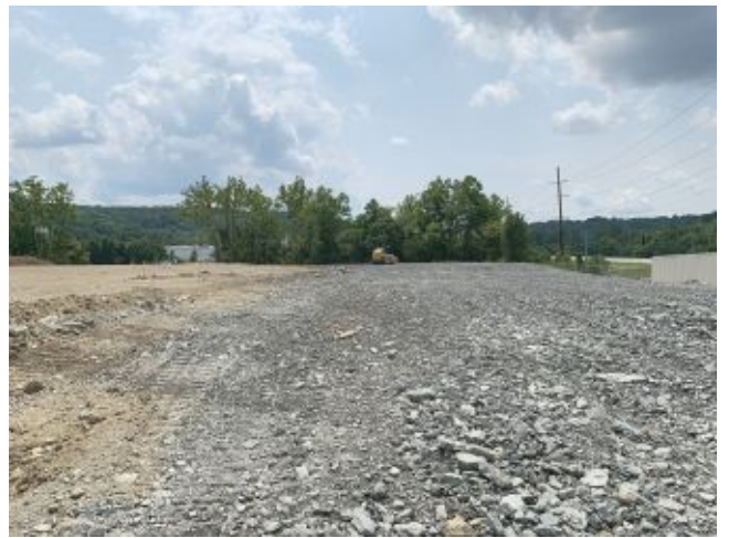
2024.07.23 – Site looking south.
