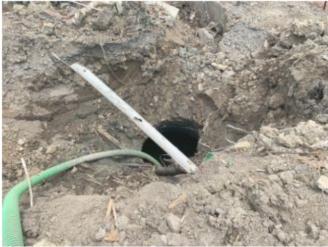
2024.06.26 – Discovered sanitary vault.
