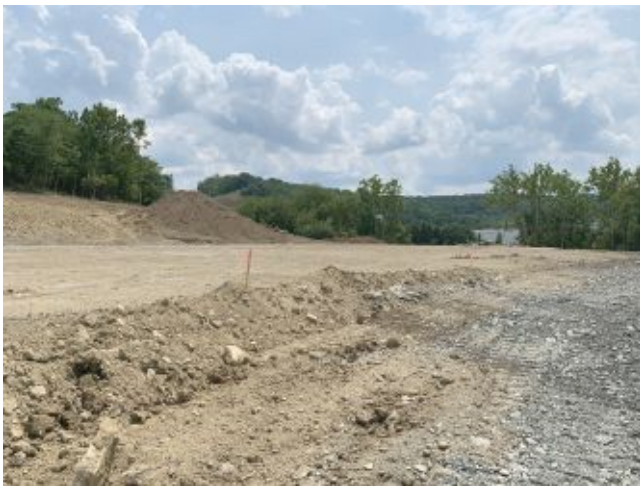
2024.07.23 – Site looking southeast.
