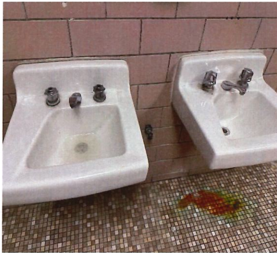
Leaking sinks, non-functioning or leaking faucets.
