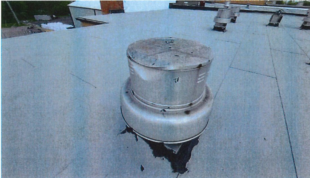
Figure 17 | Damaged Fan
