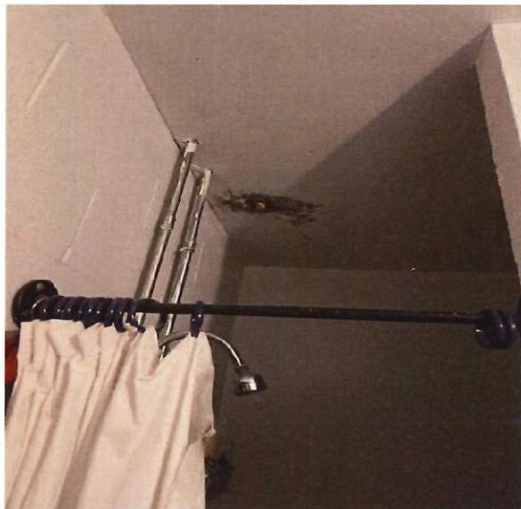
Leak above hard ceiling in the shower.
