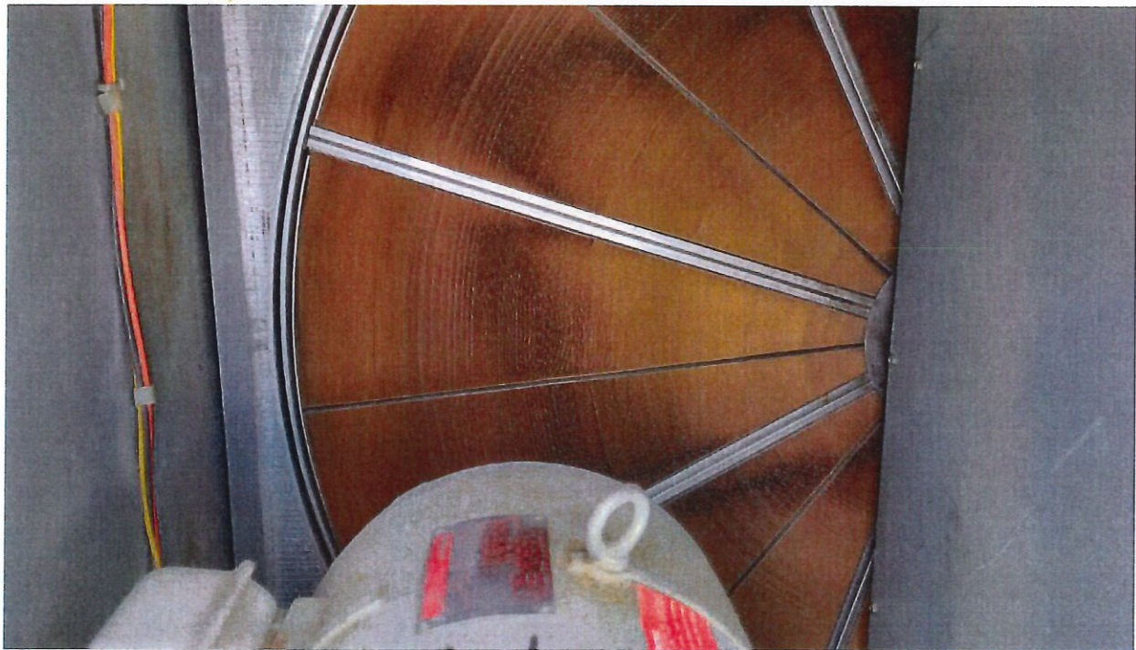
Figure 12 | The Core ERV Energy Recovery Wheel Conditions
