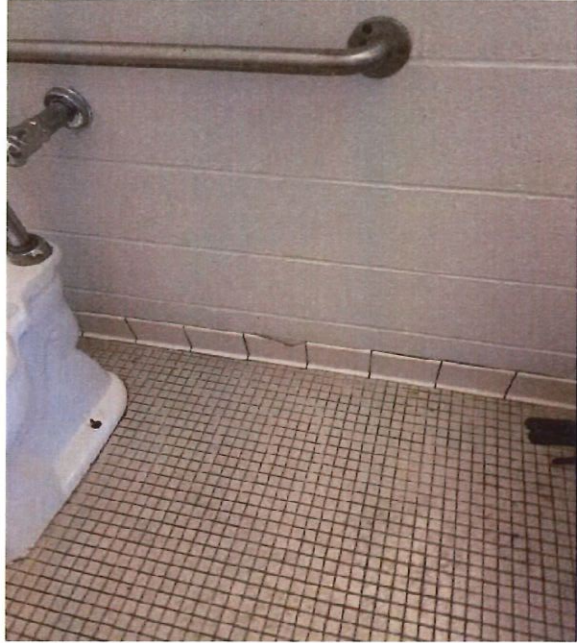
Broken or Chipped tile base.
