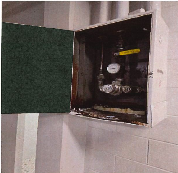
Single Valve for 8 Minimal functioning shower heads.
