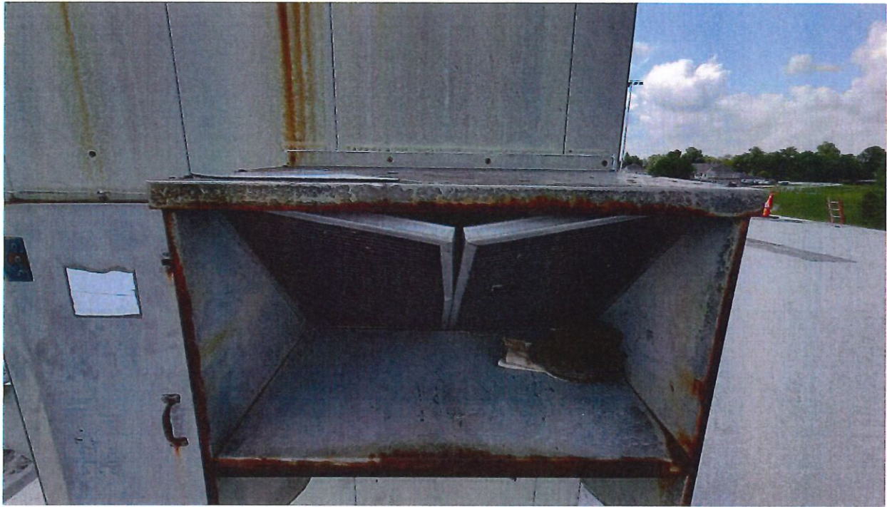
Figure 11 | The Core ERV Intake Screens
