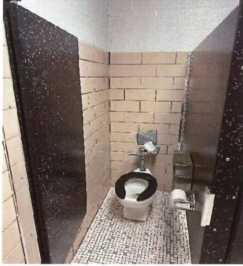
Holes behind fixtures from plumbing repairs
