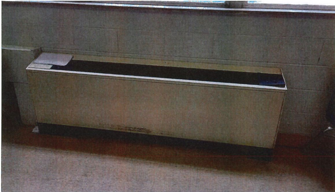
Figure 5 | The Core Fan Coils General Conditions – Installed 1997
