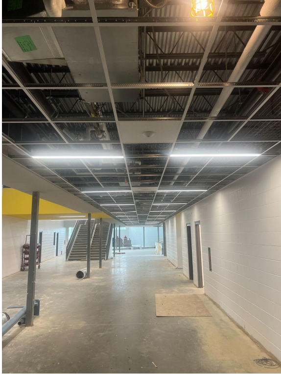
1st Floor Corridor
