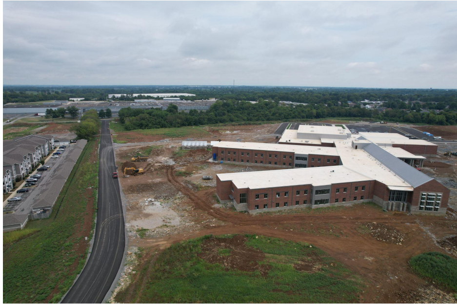
Tyrone Pike - School House Rd. Connection
