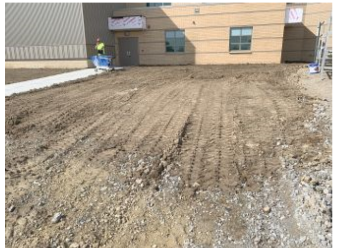
2024.05.01 – Grading East of Auditorium
