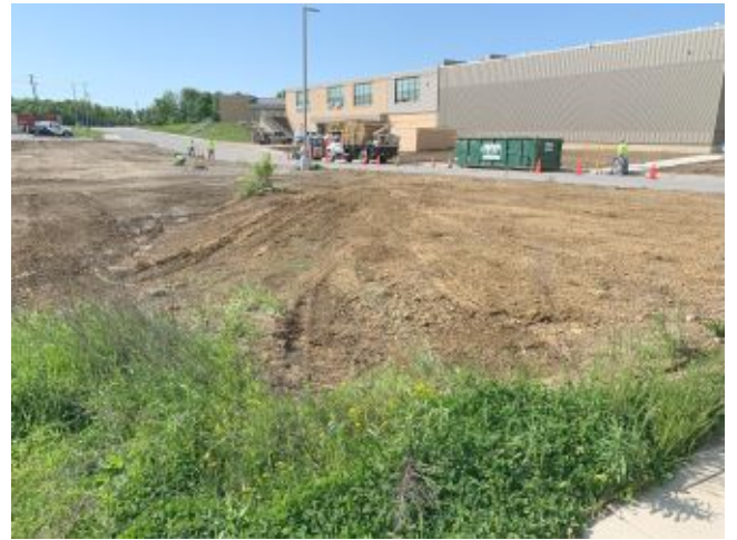
2024.05.01 – Grading East of Auditorium
