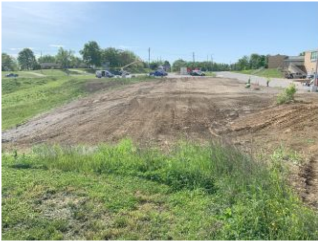
2024.05.01 – Grading East of Auditorium
