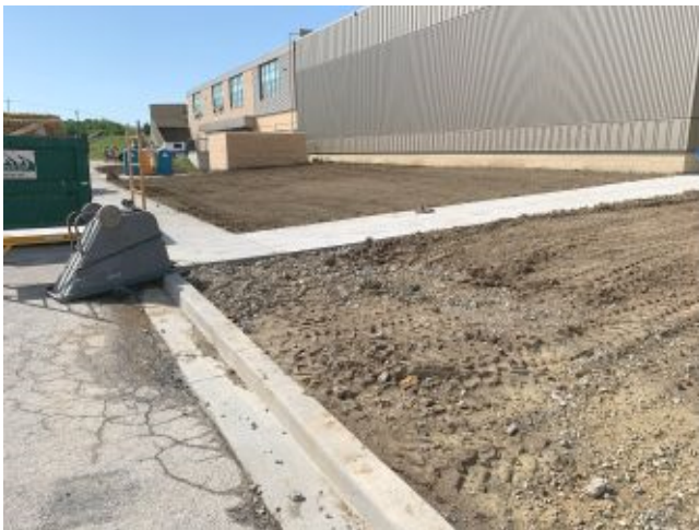
2024.05.01 – Grading East of Auditorium
