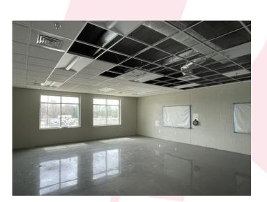
Area B (in partial) has passed above ceiling inspection for Lower Level, 1<sup>st</sup> floor, and 2<sup>nd</sup> floor. Installation of Ceiling tiles is ongoing.
