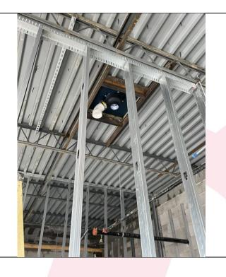
Roof drain in Area F. The roof drains in Area F need to be tied in as soon as possible for the roofer to continue his work.
