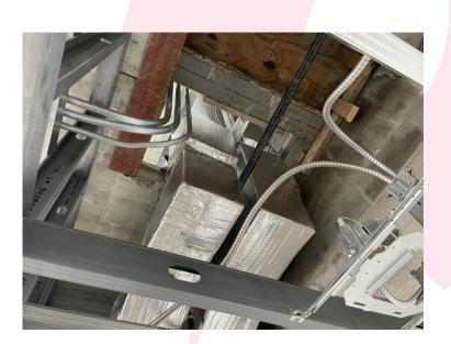
Photo of ducts penetrating the Second-floor slab in Area B. Note that the opening provided for the ducts is much larger than necessary. While the ducts do have the required fire-dampers, the remaining opening will need to be closed in via a shaft wall to maintain the 2 hour firerating. <u>Access to the fire dampers</u> must be maintained per code.
