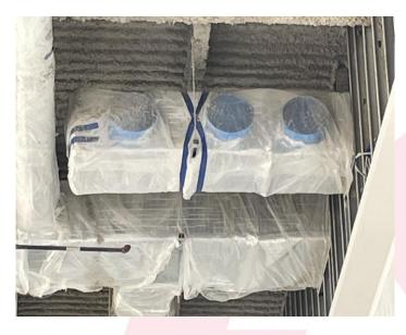
Installation of rigid ductwork in the Media Center and the Café is complete. Photo of the ductwork in the Media Center. Note that the ductwork has been wrapped with plastic to protect it from fireproofing of the structure overhead.
