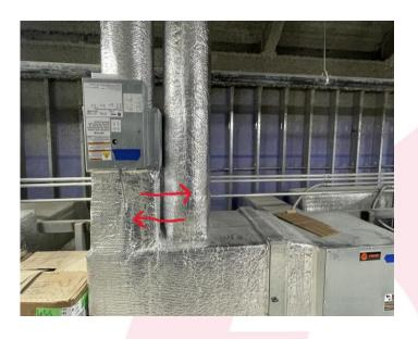
Photo shows an example of takeoffs for VAV Outside Air and Exhaust Air being installed backwards. In this installation the Outside Air will be pulled through the Exhaust Air duct, instead of reaching the spaces served.
