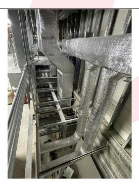
Insulation of ductwork has maintained pace with duct installation. Photo of insulated duct from the platform to below.
