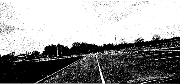
Picture # 9 View of Asphalt Looking South
