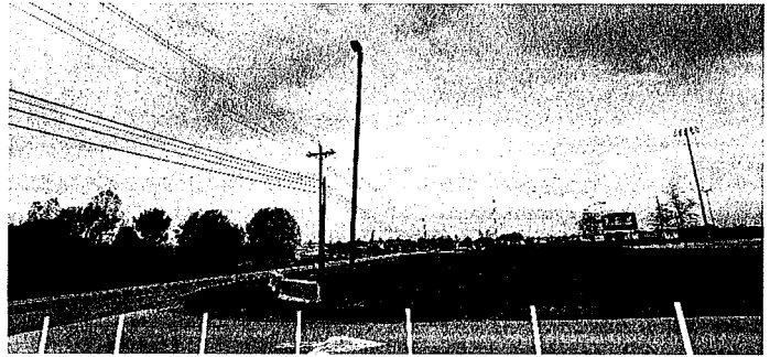
Picture # 8 View of a light pole acquired (SW)
