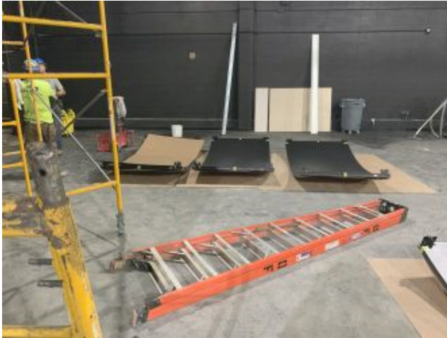
2024.03.06 – Acoustical clouds staged for installation
