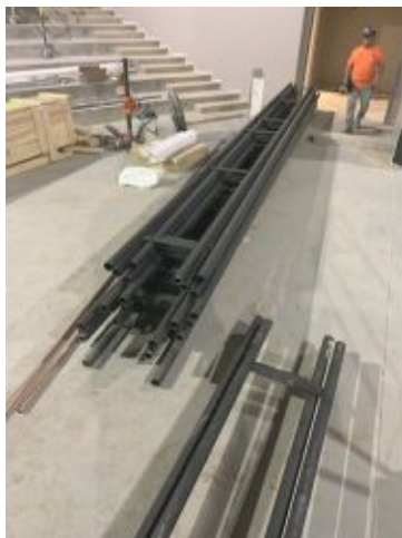
2024.02.07 – Rigging trusses / battens awaiting installation
