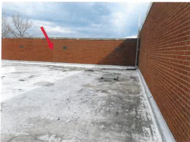
Wall receiving metal panels
