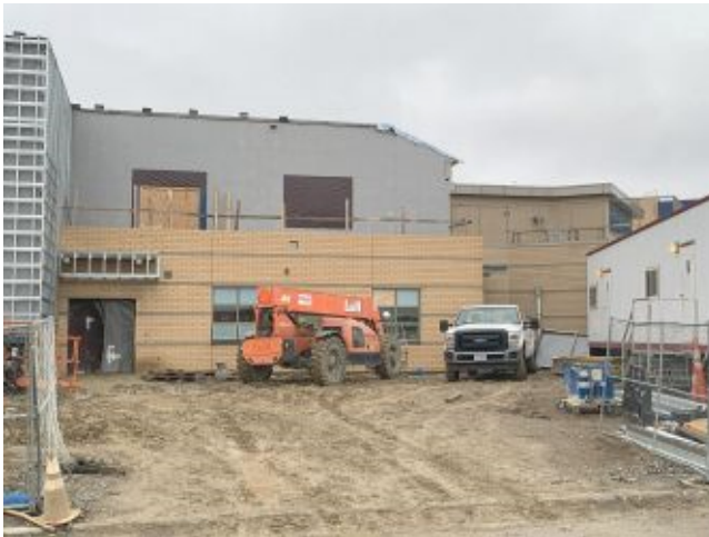
2024.01.10 – Exterior of admin addition
