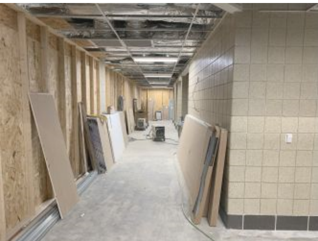
2023.12.28 – Non-occupied side of Corridor #1000C
