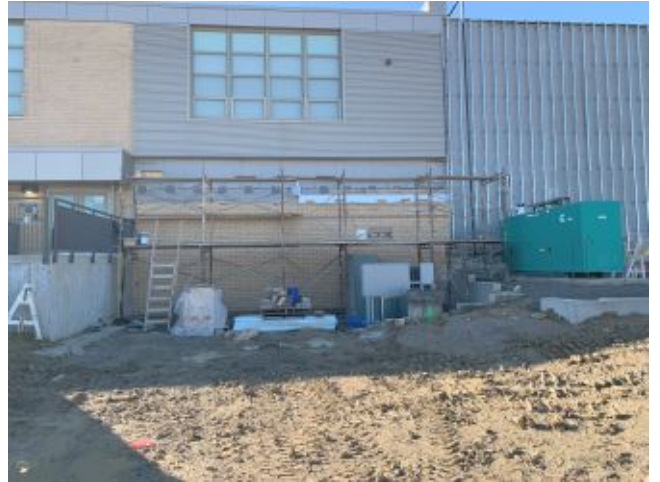
2023.12.28 – Exterior side of Green Room
