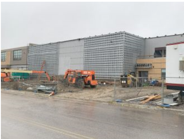
2024.01.24 – East wall of Auditorium
