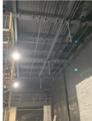
2024.01.24 – Rigging work backstage
