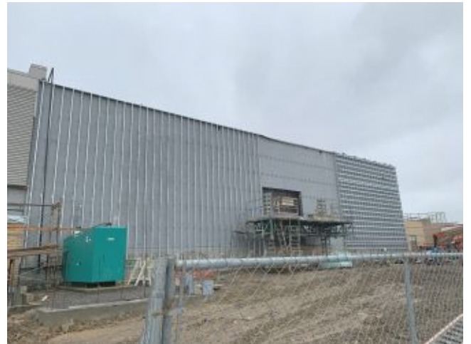
2024.01.10 – East wall of Auditorium
