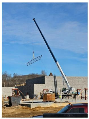
The new Calvary Elementary received the ceiling joists as well as masonry and electrical rough-in throughout the building.
