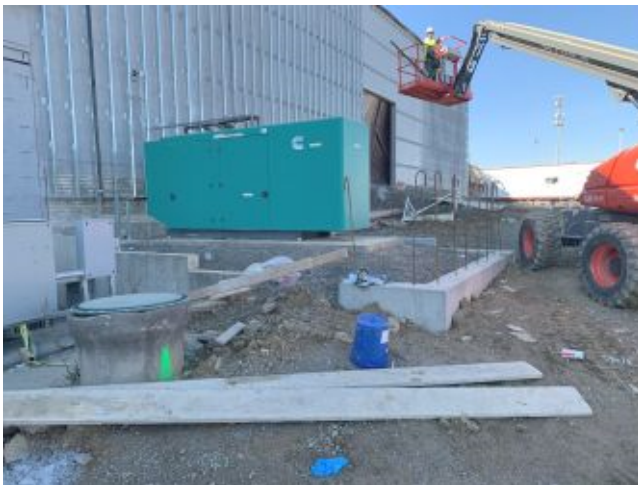
2023.12.13 – Screen wall foundations
