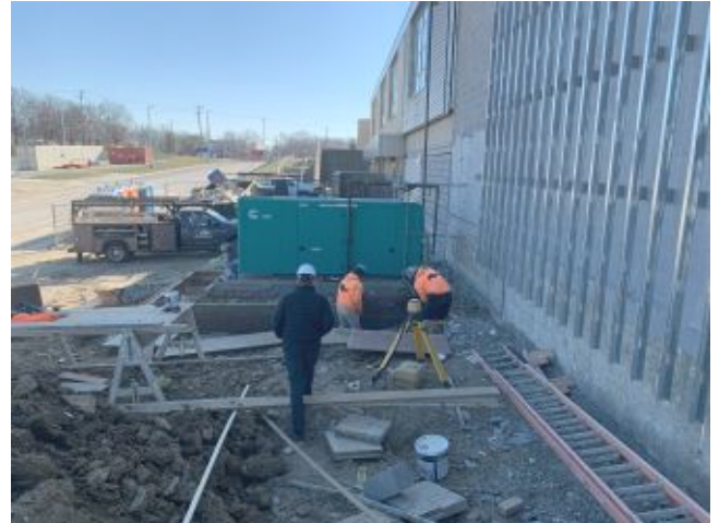
2023.11.29 – Generator foundation work
