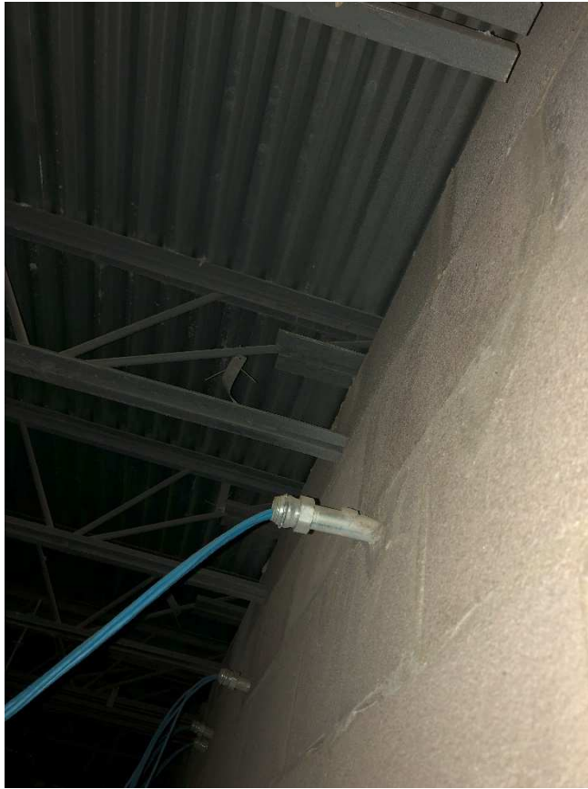
Joist bearing. No apparent issues at bearing locations observed.
