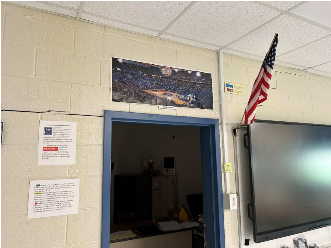
Room 131, cracks in CMU wall.
