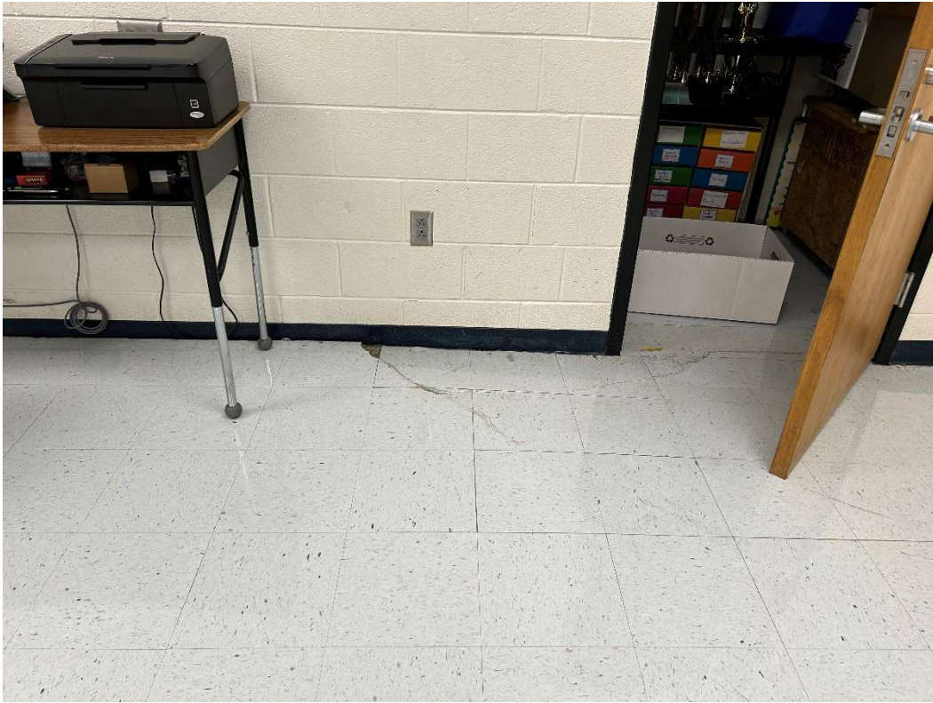
Room 121, visibly different elevations between door area and surrounding slab.
