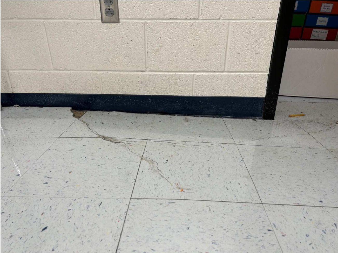
Room 121, visibly different elevations between door area and surrounding slab.
