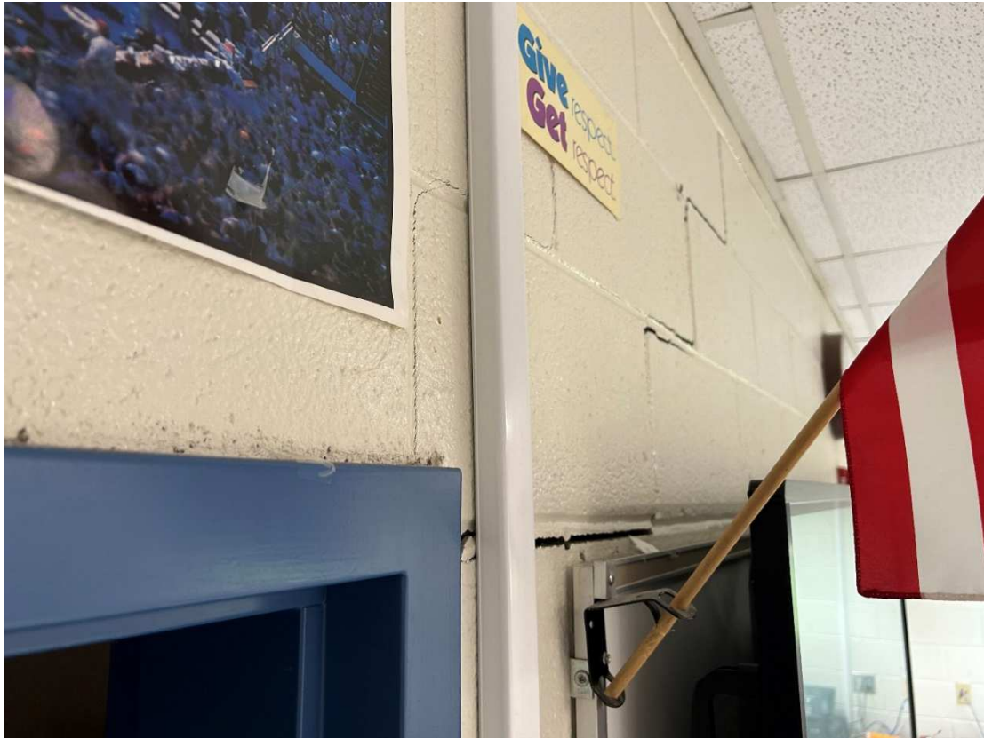
Room 131, cracks in CMU wall.
