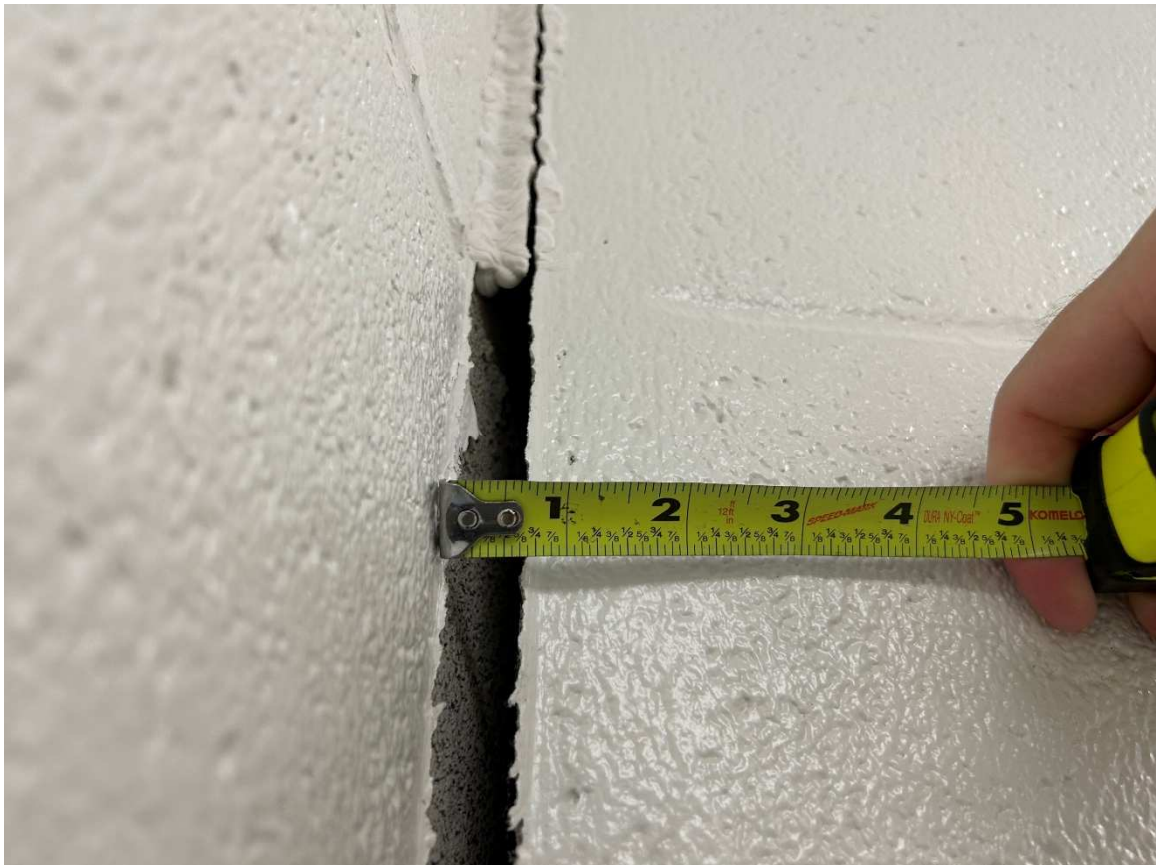
Room 119, visible gap in CMU wall (approx \frac{3}{4} " ).
