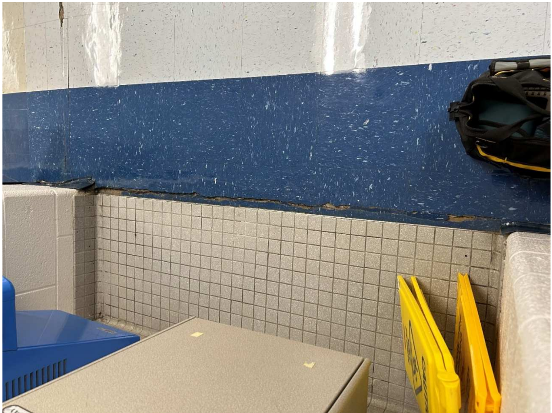
Crack in slab at water fountain (near Room 119)
