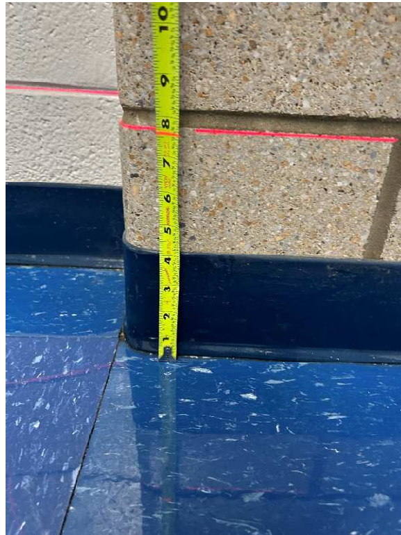
Laser level establishing reference point at front pilaster mortar joint
