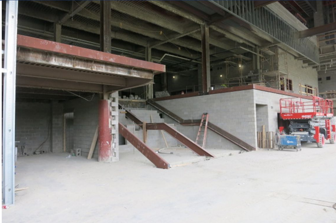
Steel at Social Stair
