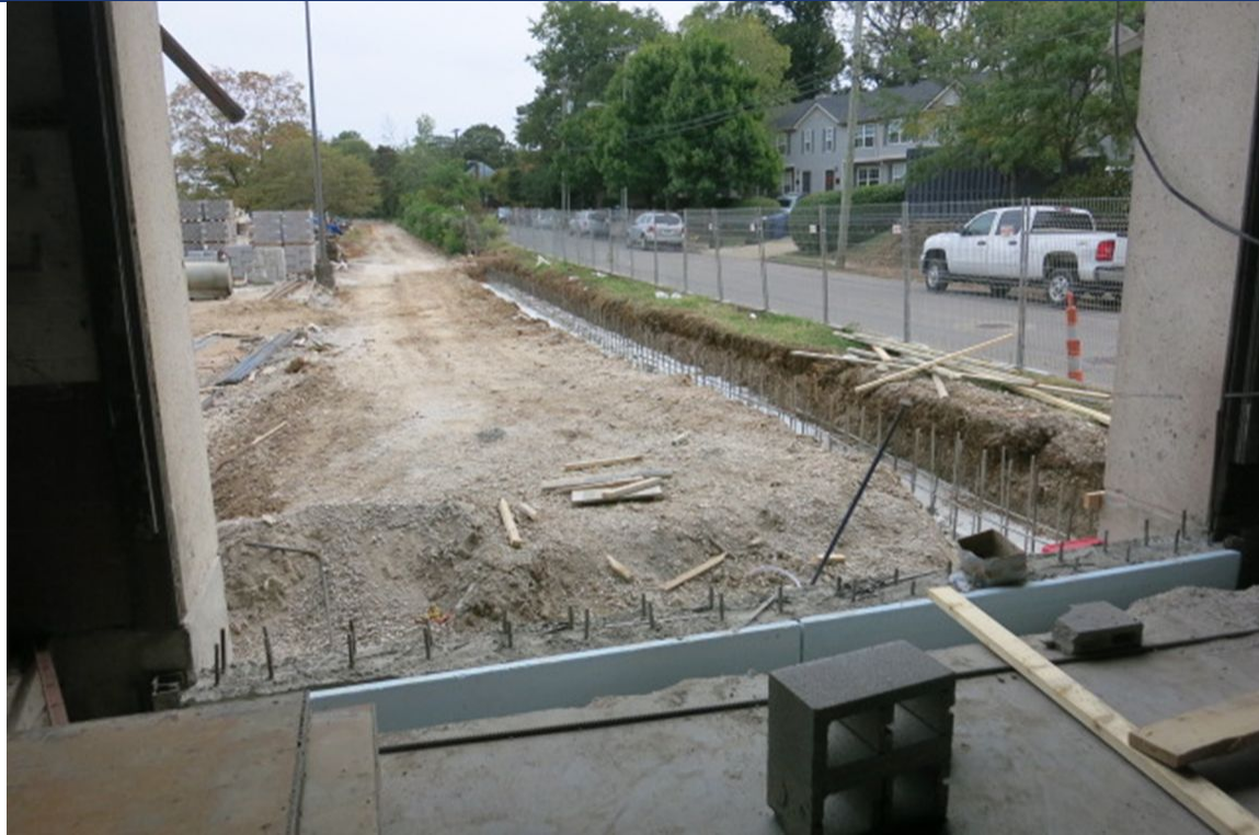
Retaining Wall Footing at Ramp
