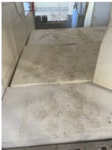
2023.09.20 – Foam fill blocks in Passage #1040C.
