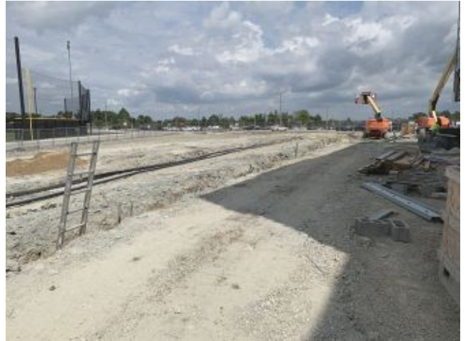
2023.09.06 – Geothermal well field under future parking lot.
