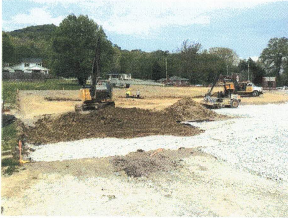
Undercutting black unsuitable fill
