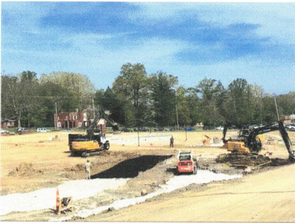
Type IV Geofabric placed for undercut
