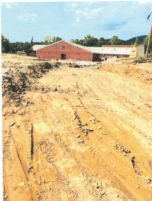
Areas failed proof roll Parent Drive
