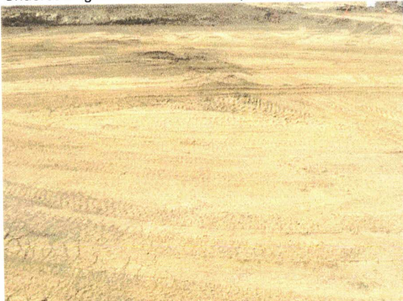
SG puming and rutting 1 ft
