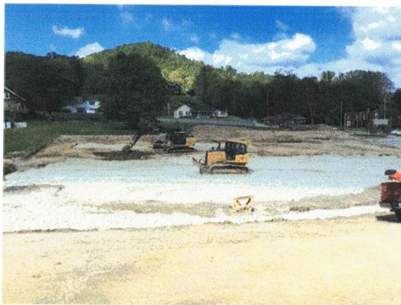
#2's being spread out with bulldozer
