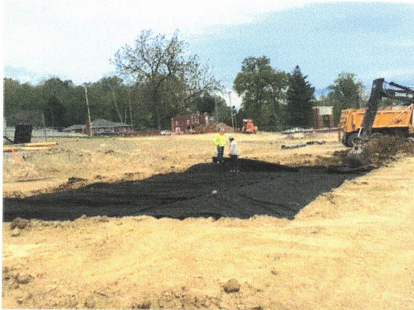
Placing of filter fabric over NW corner undercut
