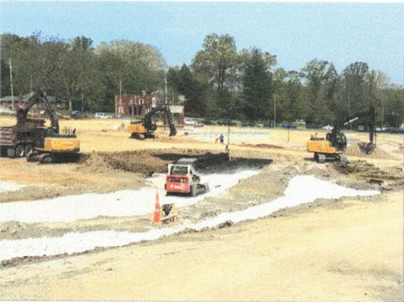
#2KYSTONE being placed for undercut
