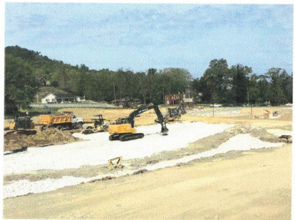
"Walking in" #2 KYSTONE with a Deere 310 Trackhoe
