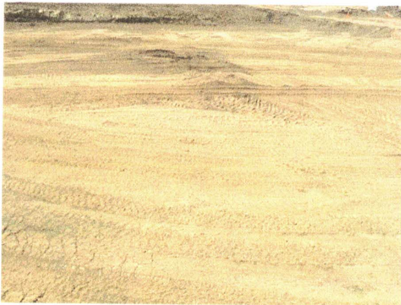
Cracked and pumping SG requiring undercut
