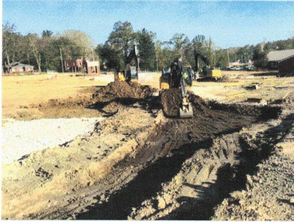
dark soil requiring 18" of undercut
