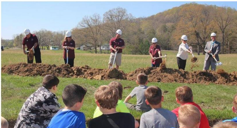
Members of the Marion County School Board put shovel to dirt at last Tuesday's groundbreaking ceremony for the Calvary Elementary School construction project. DAVID NERI / The Lebanon Enterprise
