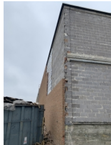
2023.03.22 – Brick veneer demolition.
