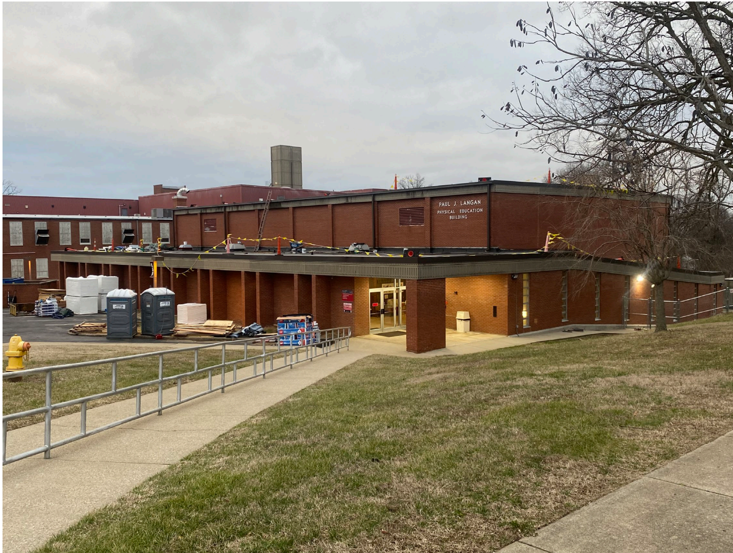
KSB Langan Gym Roof Replacement
