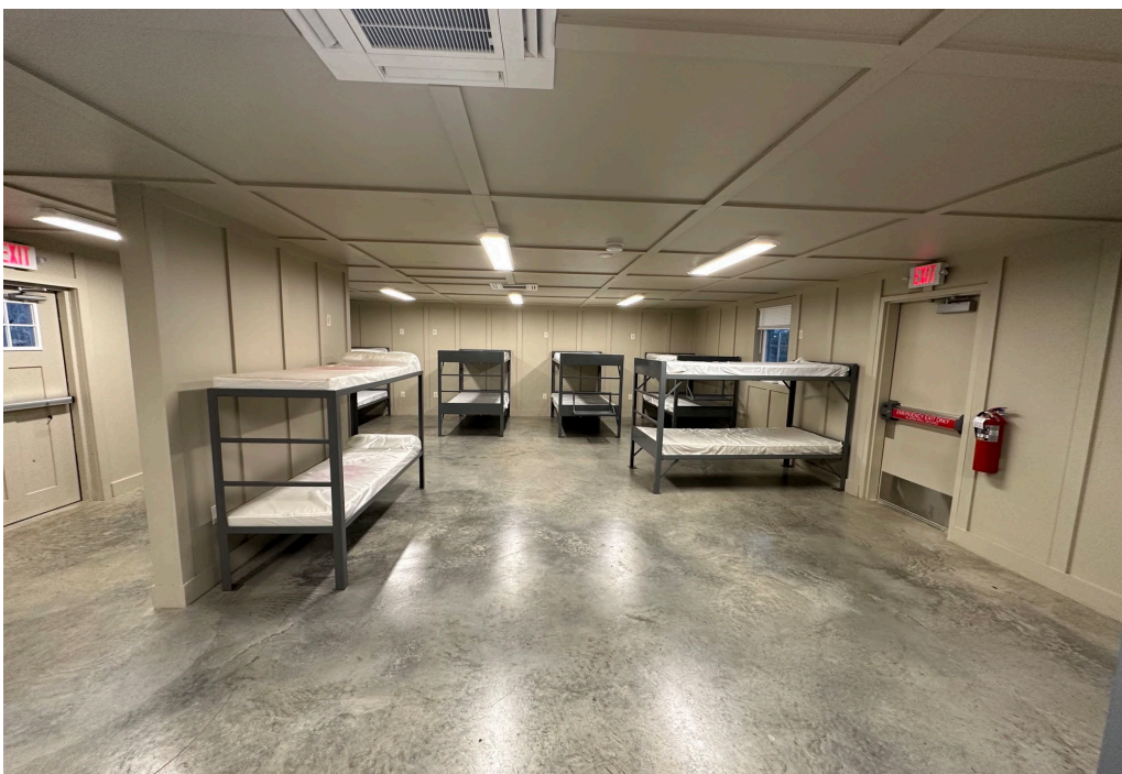
FFA Cottage Renovations
