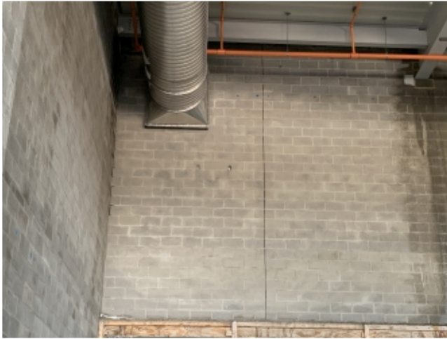
2022.12.28 – Duct transition and sprinkler pipe in pool space
