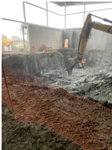
2023.01.20 – Excavation of pool deep end
