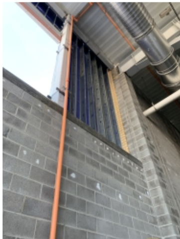
2022.12.28 PVC sprinkler pipe in pool space
