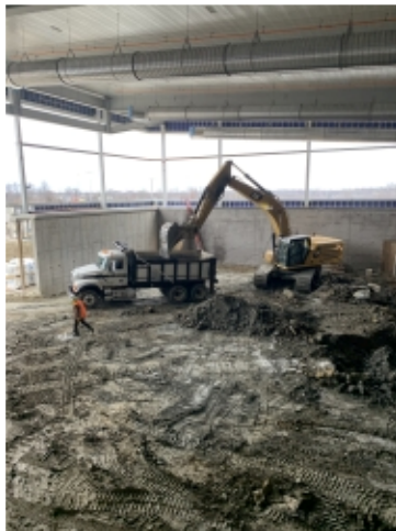
2023.01.11 – Pool excavation from above
