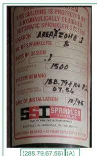
MINI AREA F" ZONE ! OF SPRINKLERS .10 1500 198.46 + 100 PS 63.59 TEGF INSTALLATION /2/96 ON . REPAIRS . 24 HOUR EMERCENCY S
