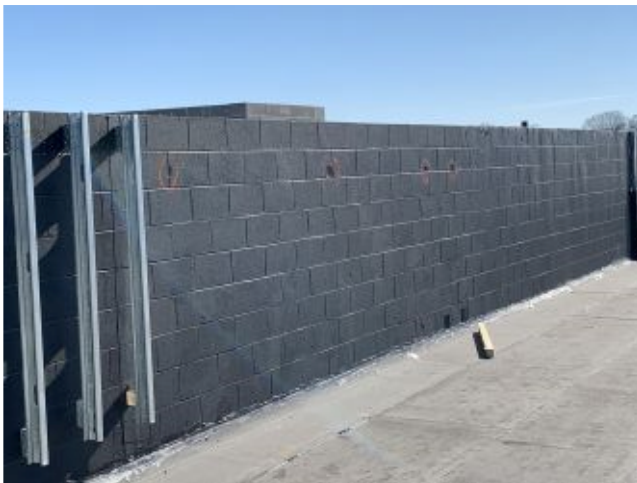
2022.11.09 – Air/weather barrier needing repair
