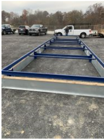
2022.11.02 – Dehumidification unit roof curb
