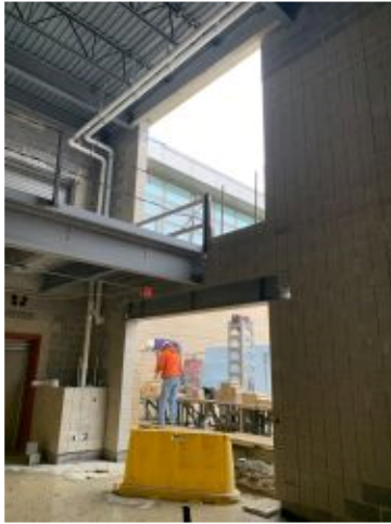
2022.11.02 – Masons working on brick veneer outside of monumental stair
