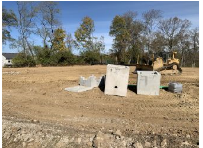
2022.10.19 – Storm structures at Taylor Mill
