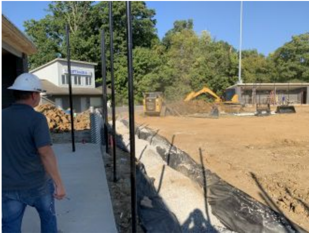
2022.09.21 – Installation of French drain
