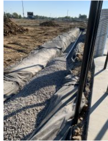
2022.09.21 – Installation of French drain
