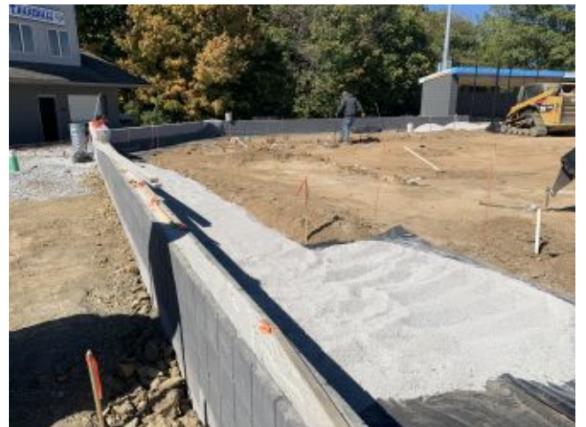
2022.10.15 – Installing warning track
