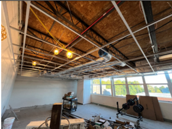
Ceiling grid installation has started.
