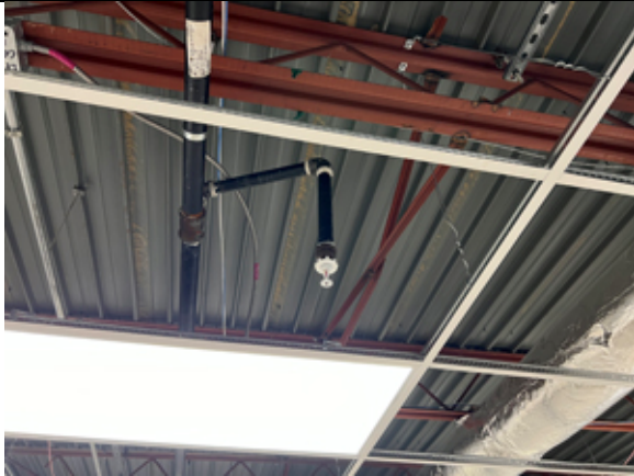
Sprinkler heads have been installed.
