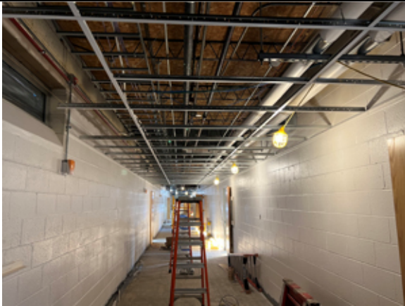
Ceiling grid installation continues throughout the second floor.
