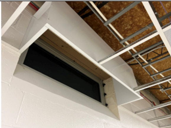
Bulkheads have been installed around the corridor windows.
