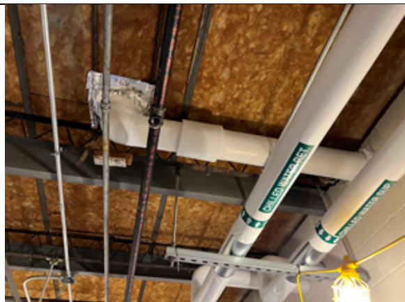
View of insulated roof drains.
