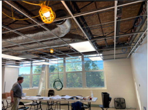
Ceiling grid installation continues throughout the second floor.
