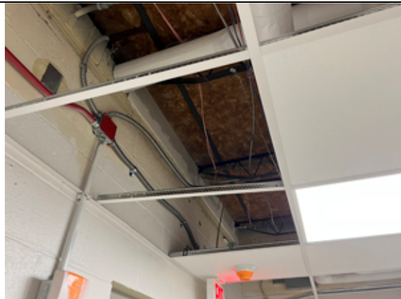
The tops of the stairwell walls have been sealed to the roof deck above.
