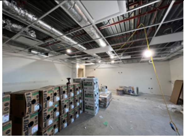
Ceiling grid installation has started.
