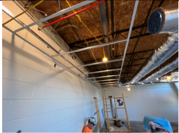
Ceiling grid installation has started.
