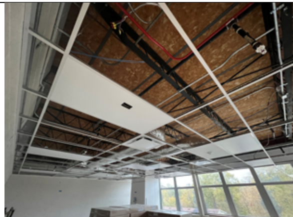
Sprinkler heads have been installed.
