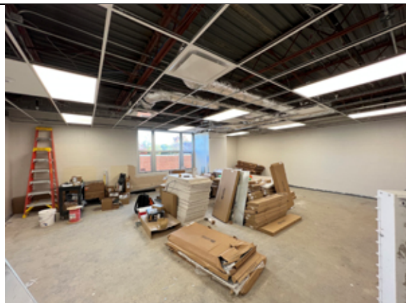
Installation of HVAC diffusers, light fixtures, and low-voltage systems continues throughout.
