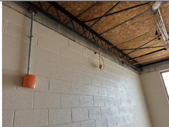
The top of the stairwells still need to be capped per the requirements of the building department.
