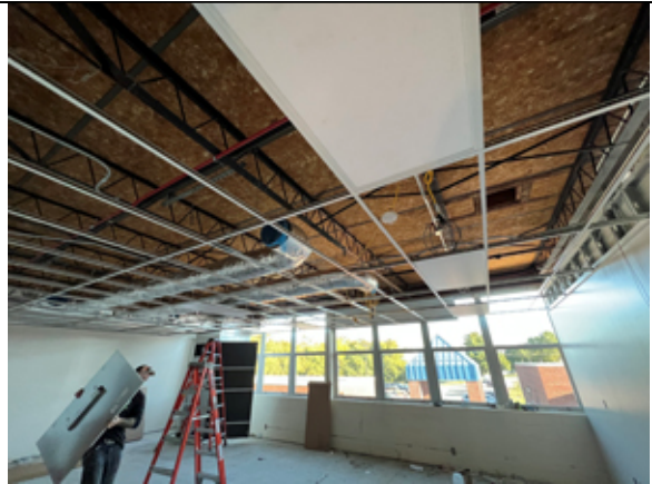
Ceiling grid installation has started.
