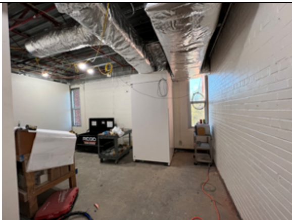
View of insulated ductwork.
