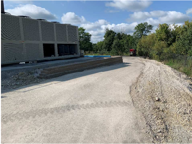
Retaining wall at chiller
