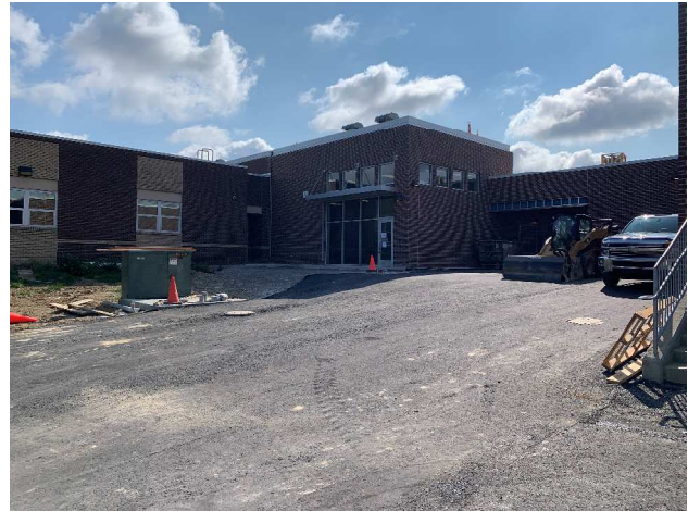
Asphalt base course at rear of building
