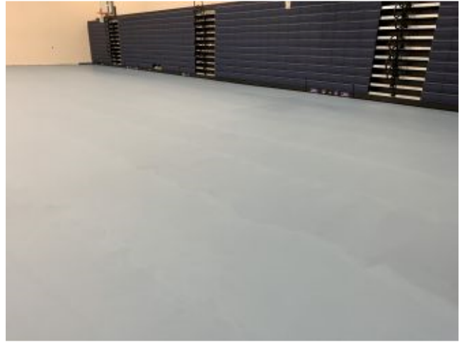
2022.09.15 - Inconsistent color at gym floor
