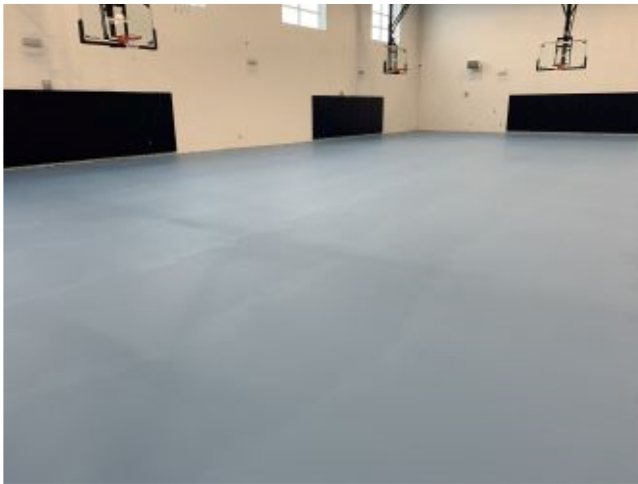
2022.09.15 - Inconsistent color at gym floor
