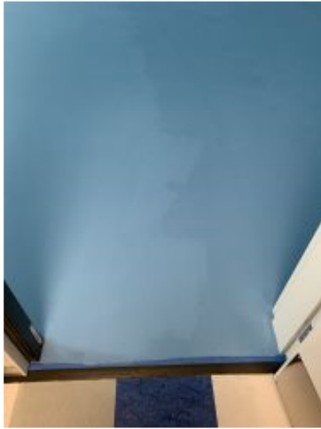
2022.09.15 - Inconsistent color at gym floor
