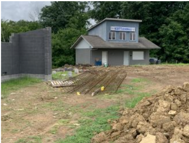
2022.08.10 – Rebar cage for rock socket at backstop net poles
