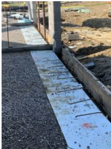
2022.07.19 – Slab insulation at pool lobby and vestibule
