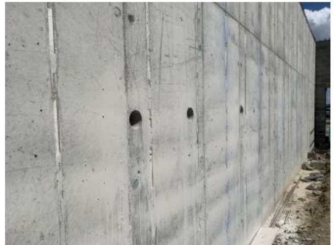
2022.08.18 – Core samples taken from pool wall
