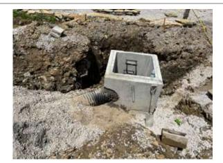
2022.07.19 Installaton of the site stormwater structures is in progress.
