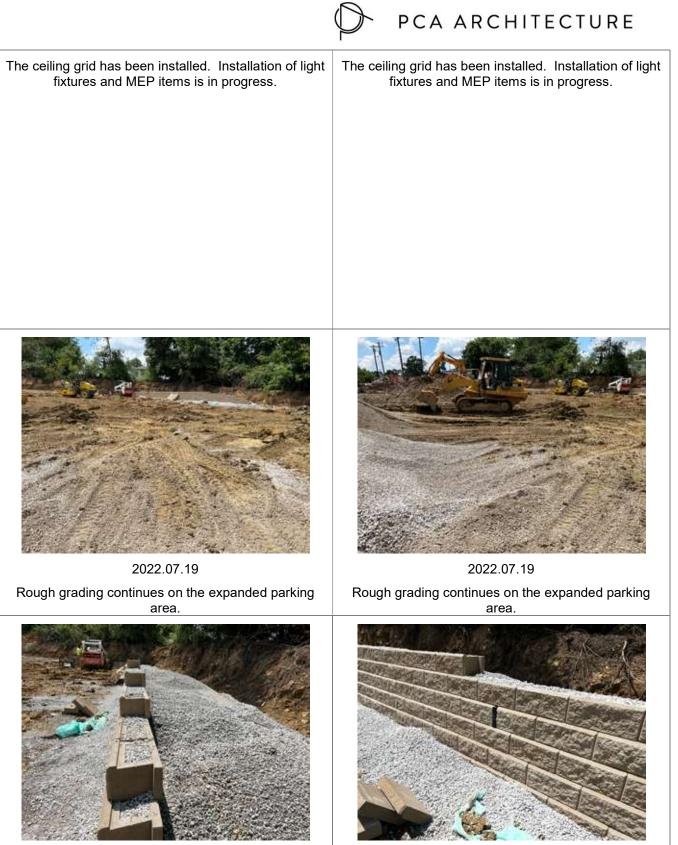
2022.07.19 Installation of the Allen Block wall is in progress.
