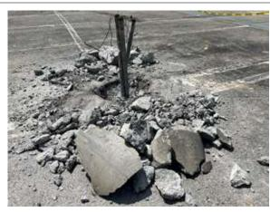
2022.08.09 Removal of the old light pole bases is in progress.
