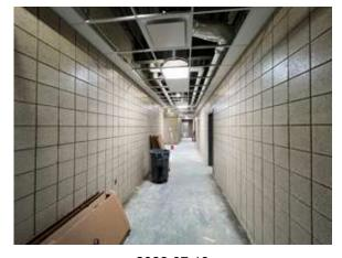
2022.07.19 The ground face cmu has been sealed. The installation of the ceiling grid and hvac diffusers is in progress.
