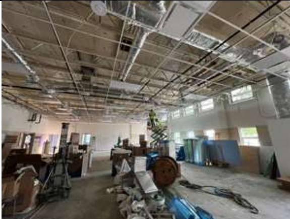
The ceiling grid for the Cafeteria is nearly complete.
