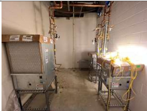
The heat pump units are being set throughout the building.
