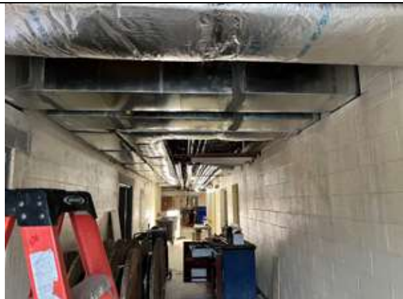
Insulation of the MEP ductwork continues throughout the building.
