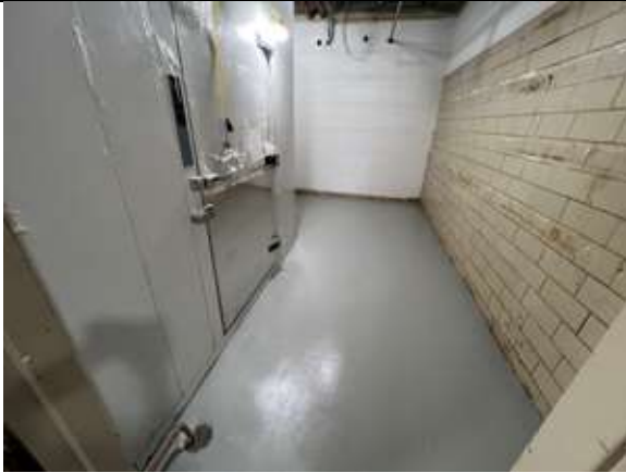
The epoxy floor has been installed in the Kitchen Storage Room.
