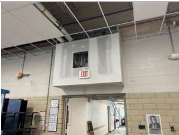
A new bulkhead has been constructed in the Cafeteria to conceal the new MEP items.
