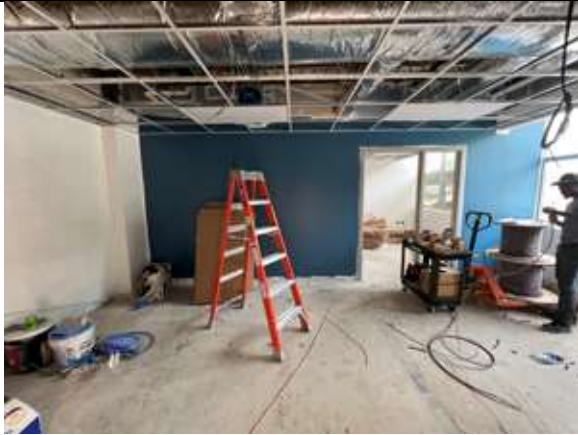
The ceiling grid has been installed in the Admin Office. Painting is in progress.
