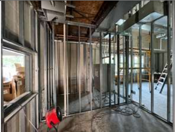
Installation of metal stud framing and MEP items is in progress in the SRO office and Faculty Lounge.
