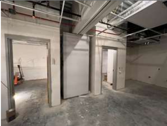
Installation of the folding partition has been completed.
