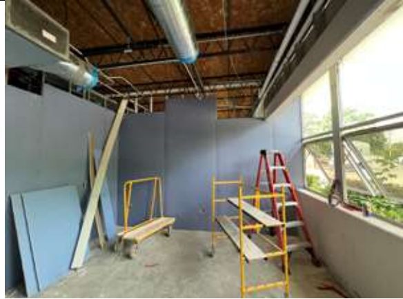
Installation of sound attenuation insulation and gypsum board is in progress in the Admin Suite.
