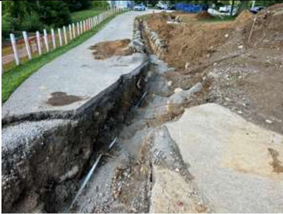
View of new water line and fire line – before trench backfill.
