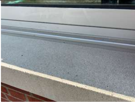
The sill flashing has been installed under the windows in the new addition.
