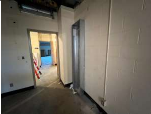
The electrical panel tub for the second floor has been set.
