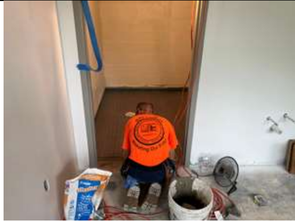
Installation of the ceramic tile in the Nurse's toilet room is in progress.
