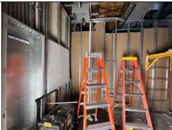
Gypsum board is being installed in the SRO office and Faculty Lounge.
