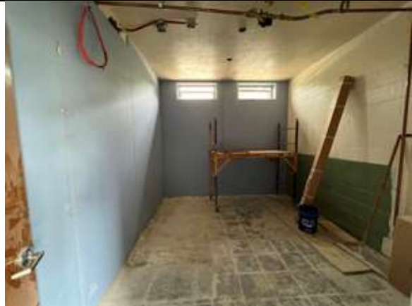
Gypsum board has been installed in the Custodial Office.
