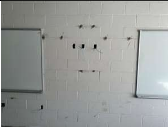
The exterior walls have been patched where the foam insulation was installed.
