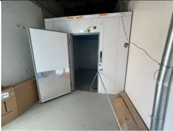
The walk-in freezer has been installed.
