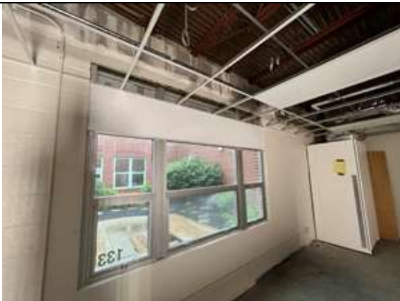
A decorative panel has been installed over the insulated metal panels installed above the existing windows.
