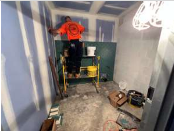
Gypsum board finishing is in progress in the Admin Suite.
