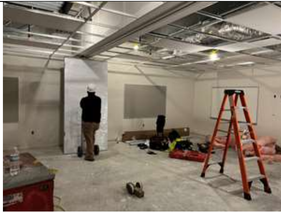
Installation of the folding partition panels is in progress.
