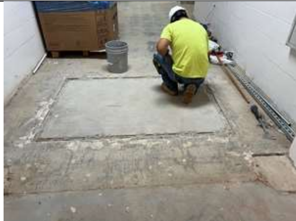
Patching of the recessed areas for the former walkoff mats is in progress.
