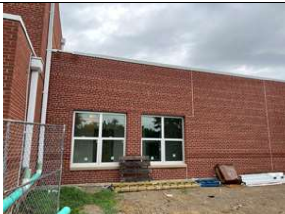
The copings have been installed on the roof. A couple areas need to be corrected and completed.
