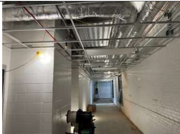
Installation of the ceiling grid continues throughout the building.
