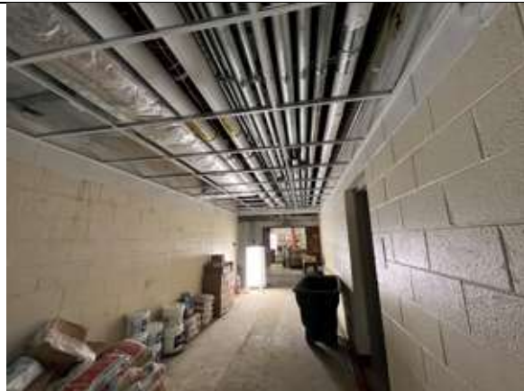
The ceiling grid has been installed in the corridors of the original building.
