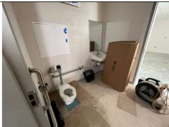
Toilet fixtures and the toilet accessories have been installed in the new toilet rooms.
