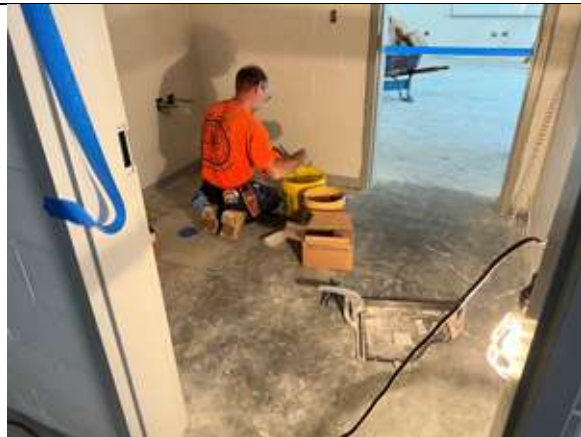
Installation of the ceramic tile in the new toilet rooms is in progress.
