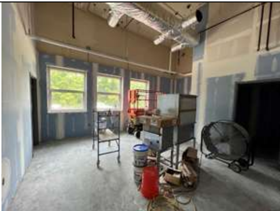
Finishing the gypsum board in the Faculty Lounge is in progress.
