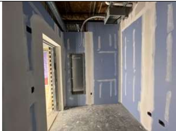
Finishing the gypsum board in the SRO Office is in progress.
