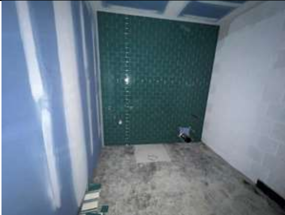
The ceramic tile has been installed on the wet wall in the Admin Suite toilet room.
