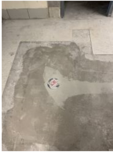
2022.07.21 – Patched slab outside of Kitchen Office
