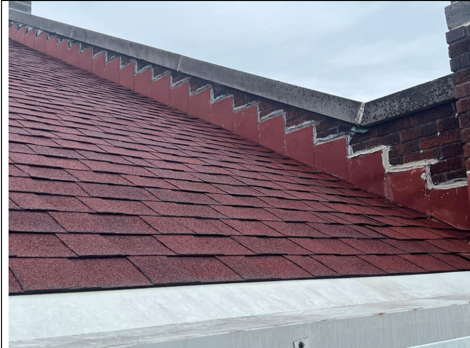
A. - Auditorium Gable Step Flashing Sealant Repairs. Both sides of gable will be repaired.
