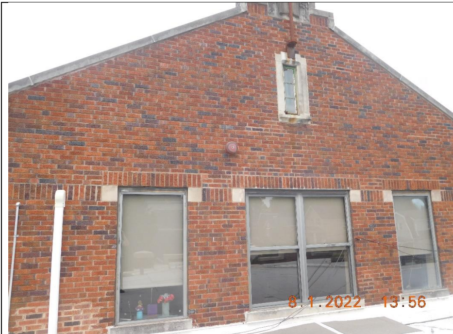
B. - Auditorium Gable End Clean & Water Repellent. Entire wall from south corner to north corner.
