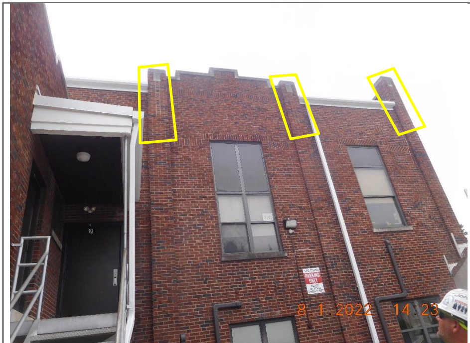
D. – North Wall Auditorium Pilaster Tuckpointing
